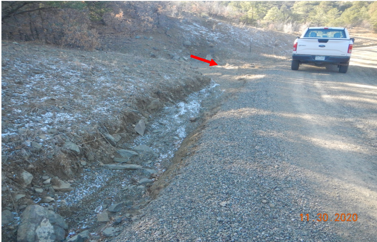
Photo 1. There is erosion along the access road and the culvert is filled in with sediment shown at red arrow.
