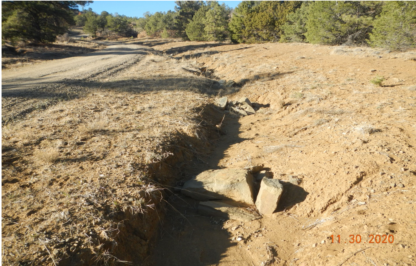
Photo 5. Facing north along the main road near the location. The side of the road has eroded. The rock check dams have failed.
