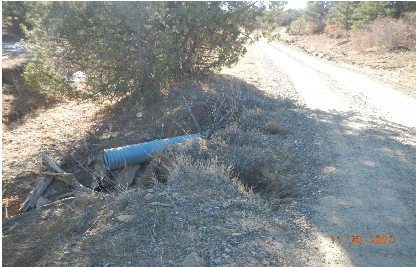
Photo 2. There is erosion at the culvert outlet at Lat/Long:37.15900,-104.81291.
