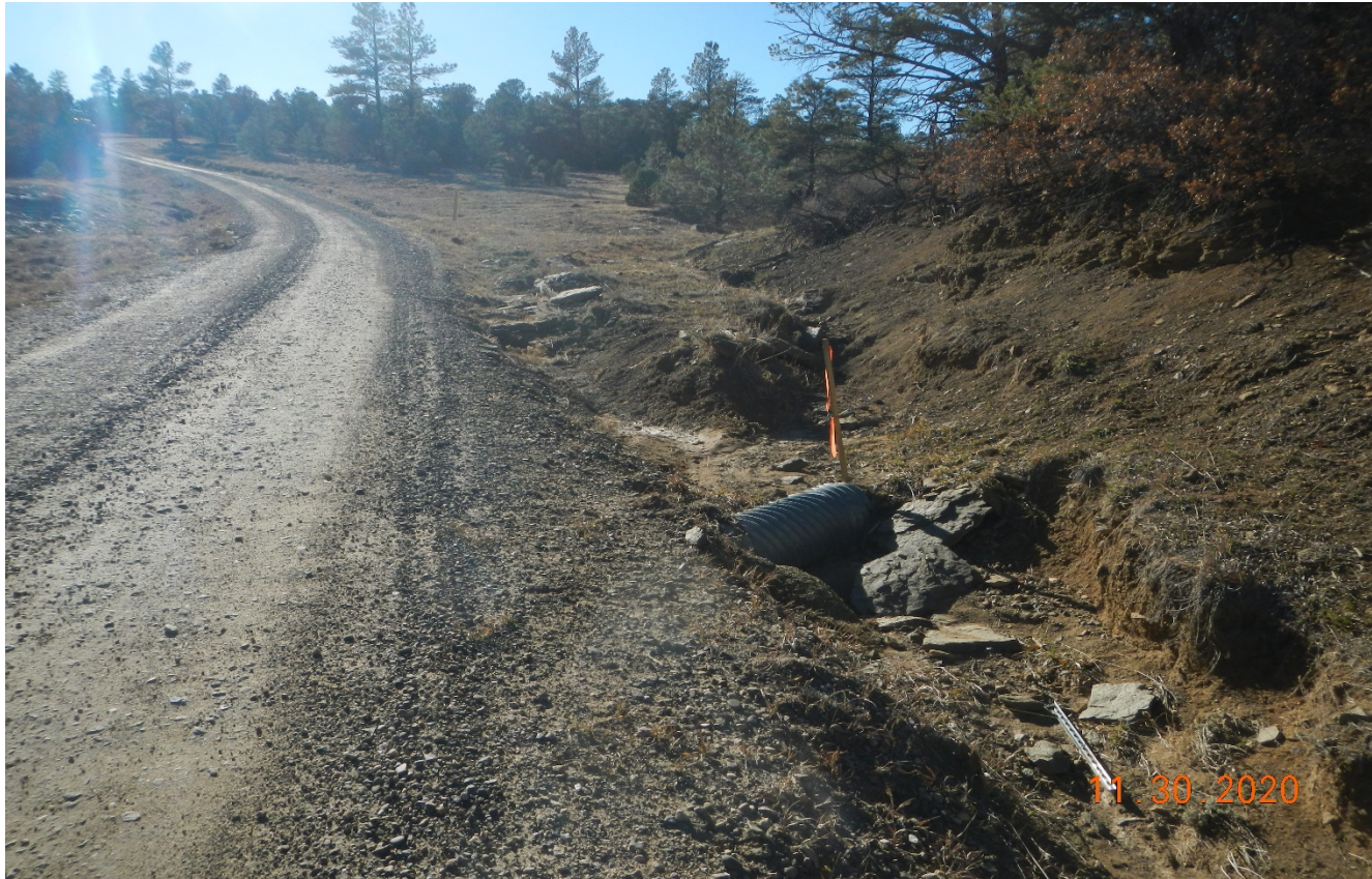
Photo 3. Facing southwest along the main road. This culvert is not maintained causing erosion along the side of the road.
