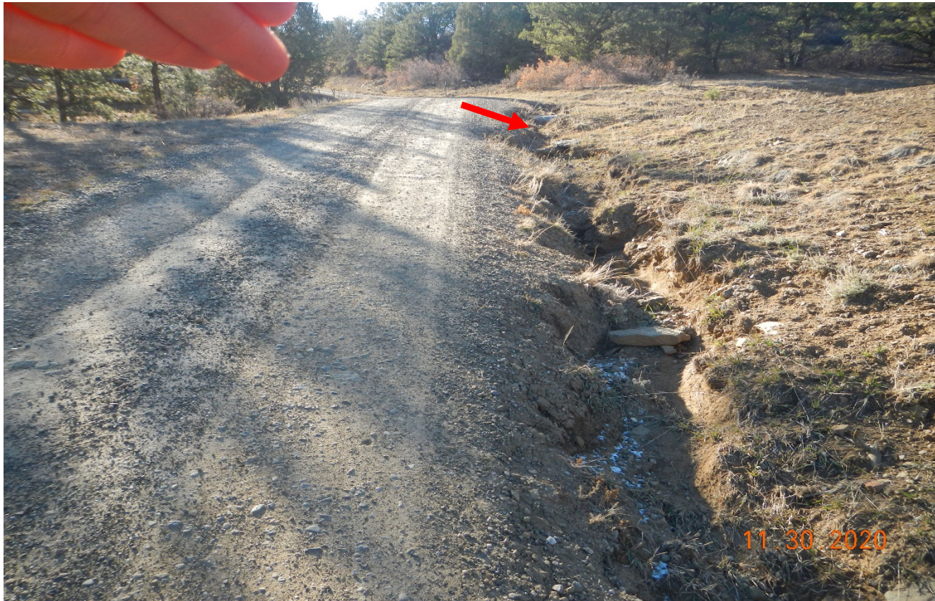
Photo 1. Facing southwest along the main road. The culvert shown at red arrow is not maintained causing erosion along the side of the road. Lat/Long:37.15900,-104.81291.
