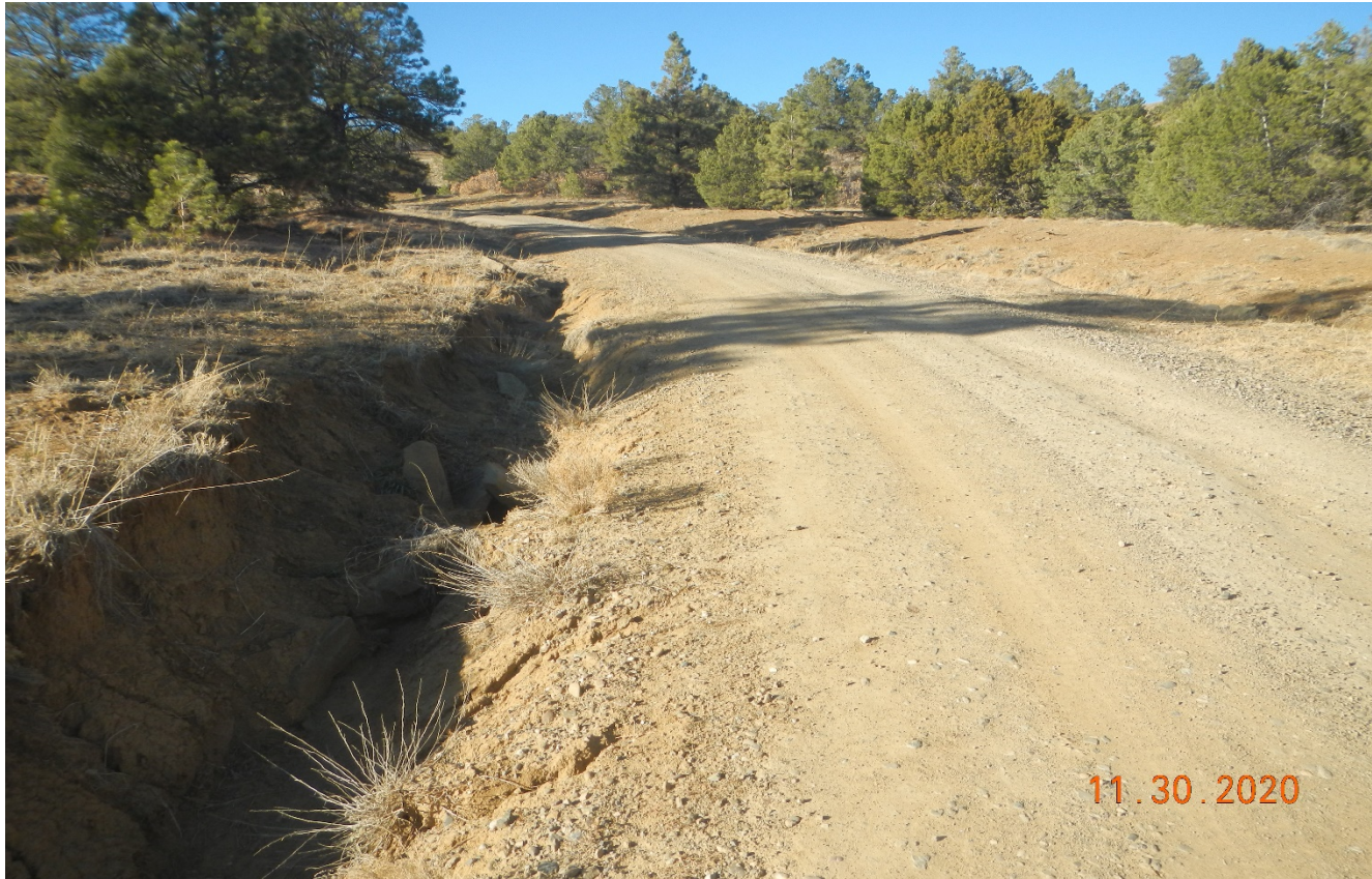
Photo 4. Facing north along the main road near the location. The side of the road has eroded.
