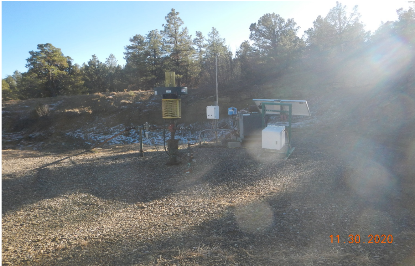
Photo 2. Facing toward the wellhead.
