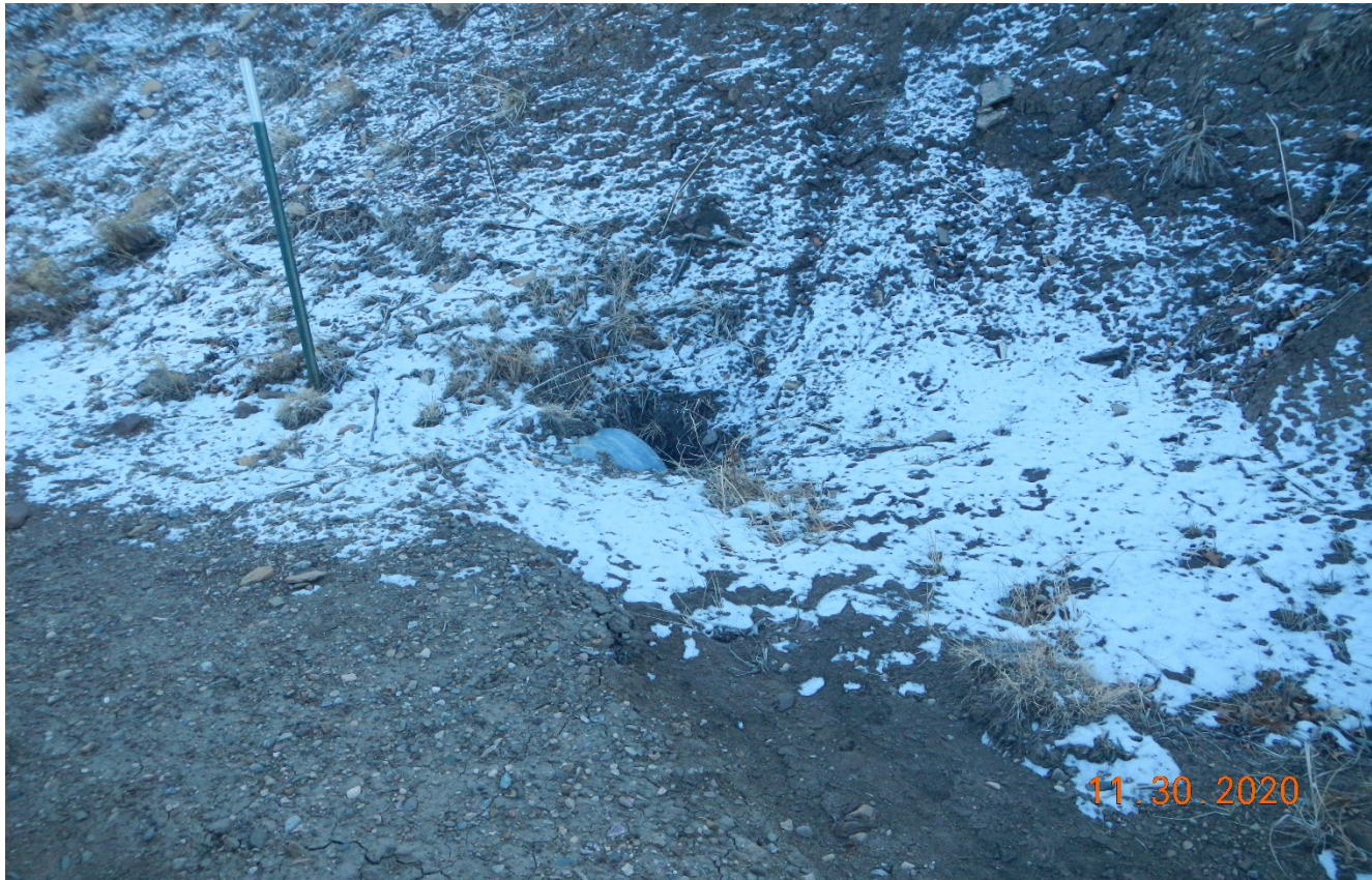
Photo 3. Culvert along the access road is partially filled in with sediment.
