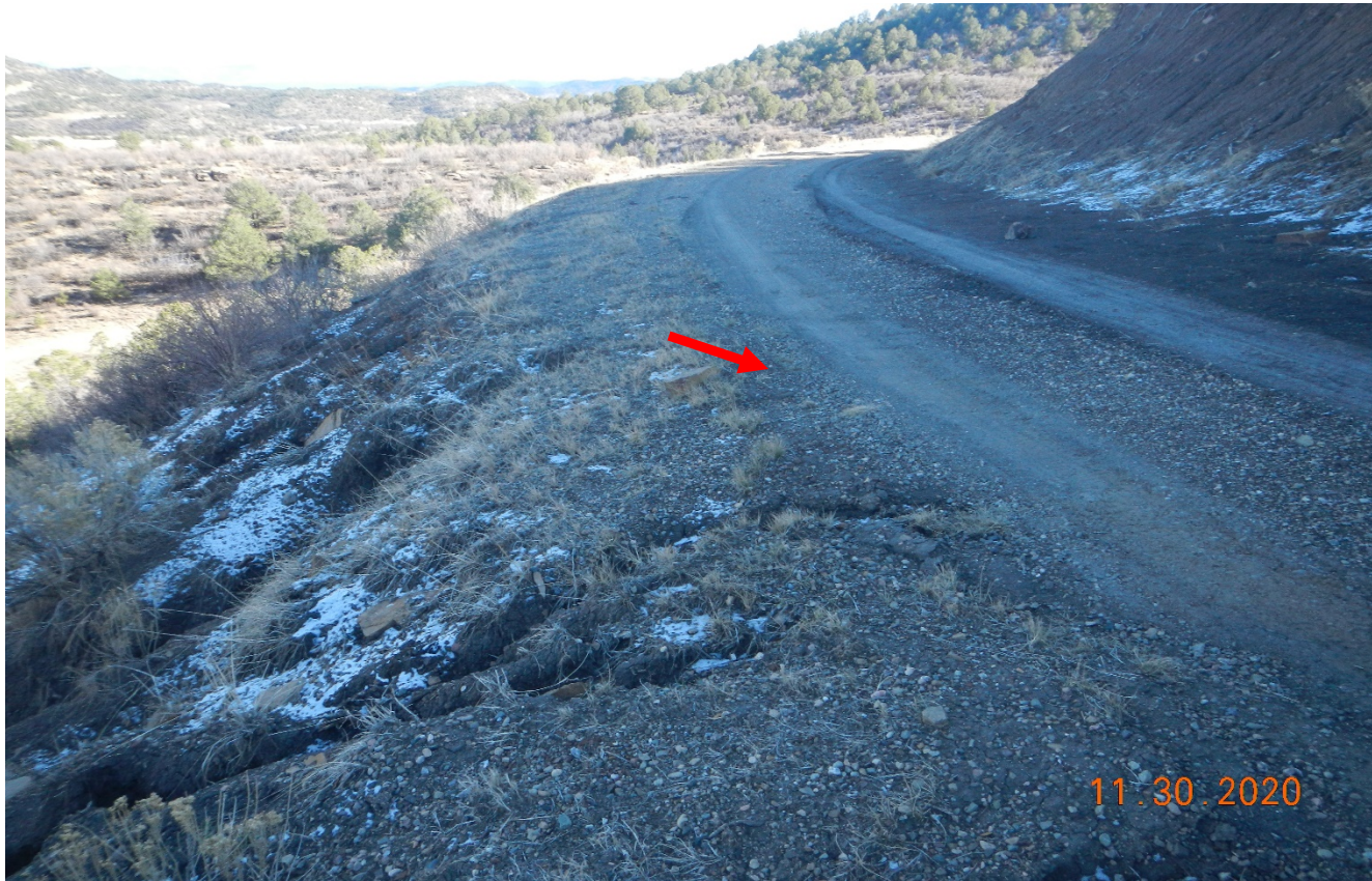
Photo 1. Facing southeast along the access road. Stormwater is directed across the road causing erosion of the fill slope.
