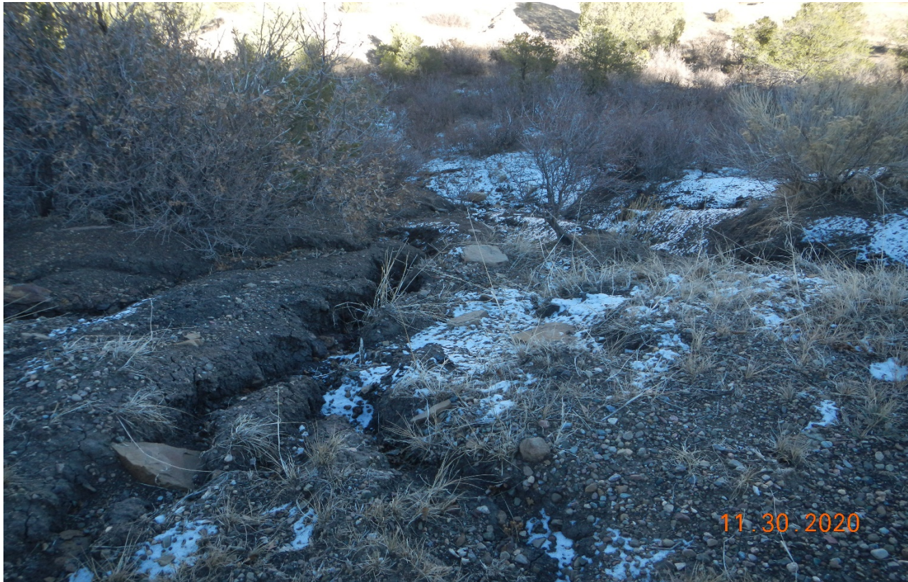
Photo 2. Facing toward the fill slope of the road showing the erosion at Lat/Long:37.14779,-104.78849.
