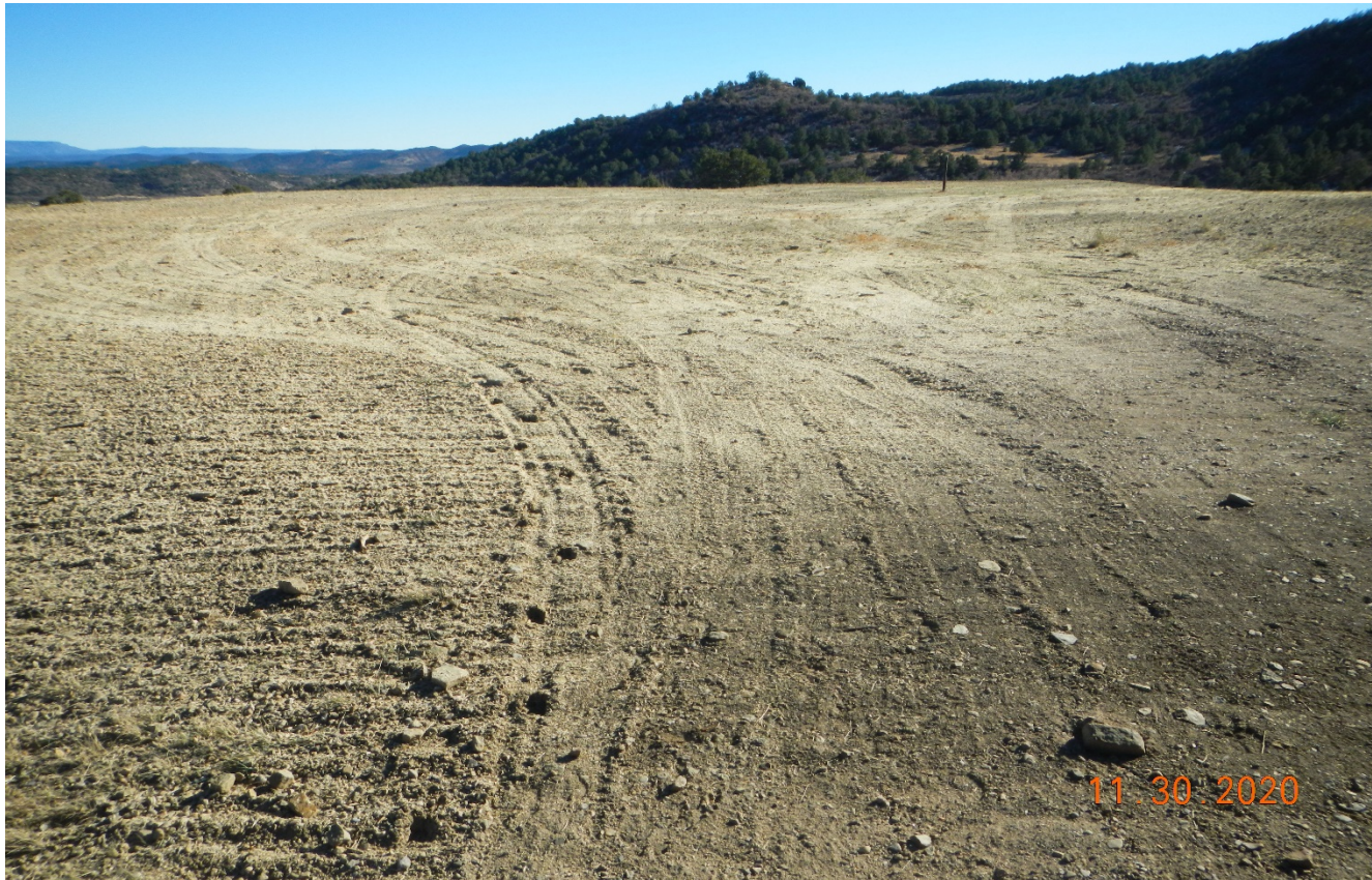
Photo 2. Facing southeast toward the location. The location has been seeded and stabilized with hydromulch.
