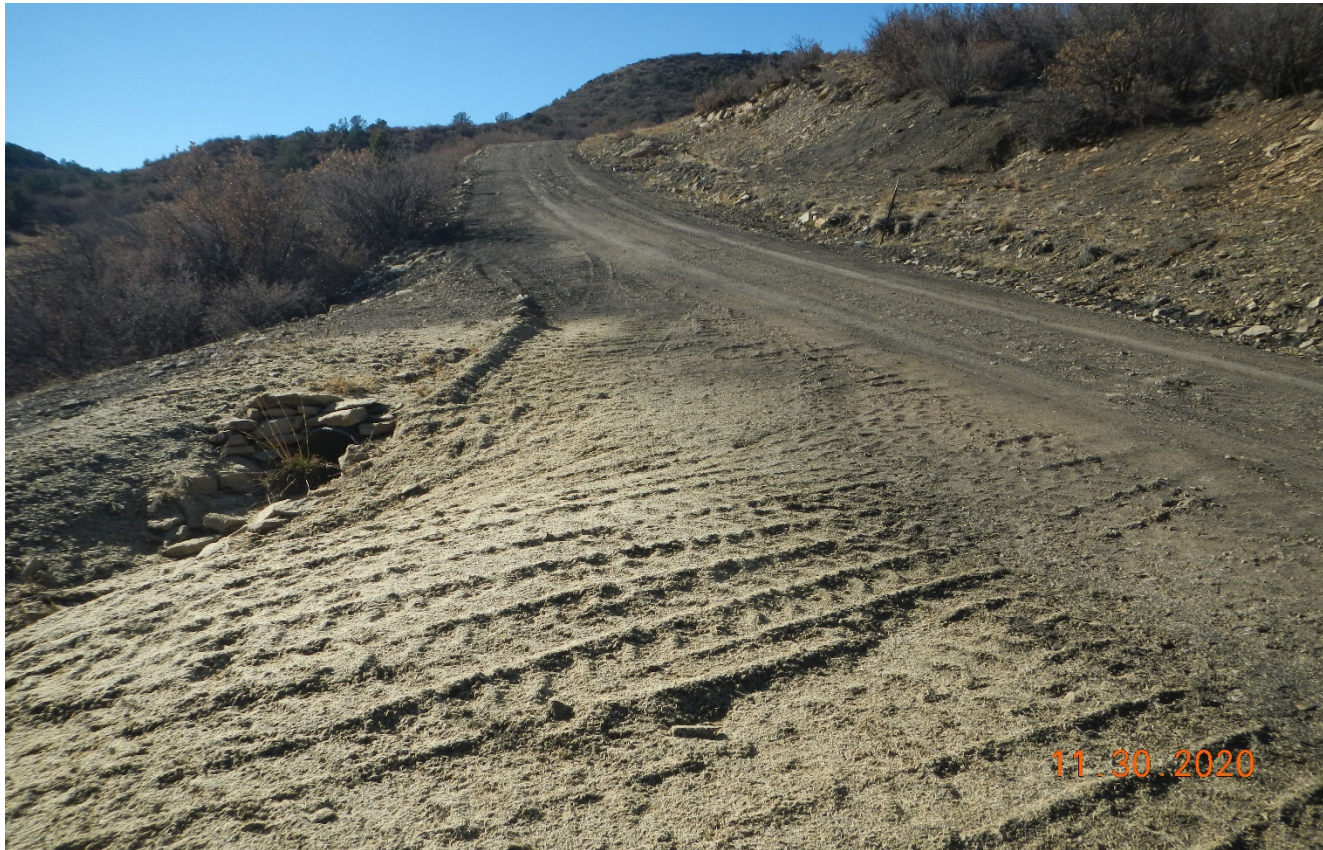
Photo 1. Facing east along the access road. Stormwater erosion has been repaired and stabilized.
