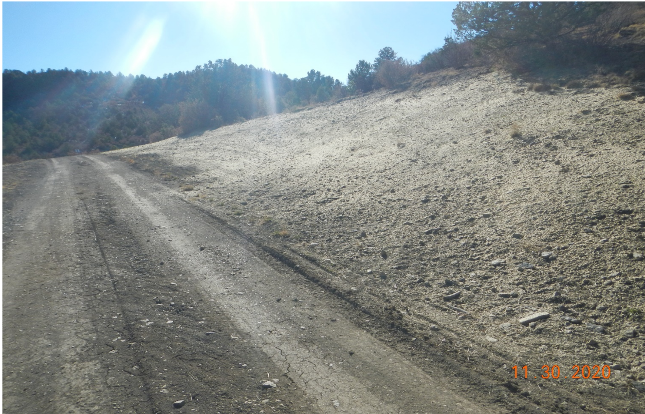
Photo 3. The cut slope has been seeded and stabilized.
