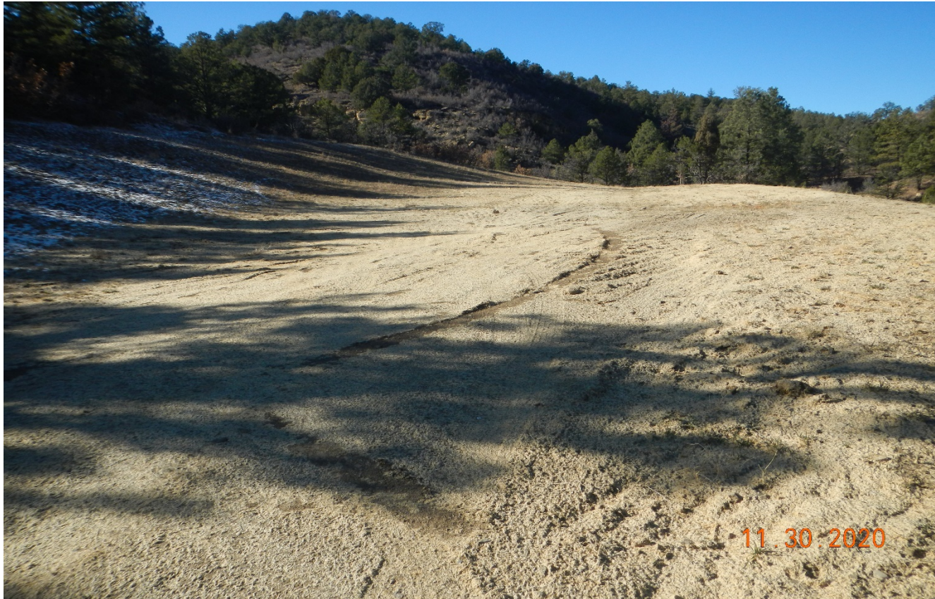
Photo 1. Facing northwest toward the location. The location has been seeded and stabilized with hydromulch.
