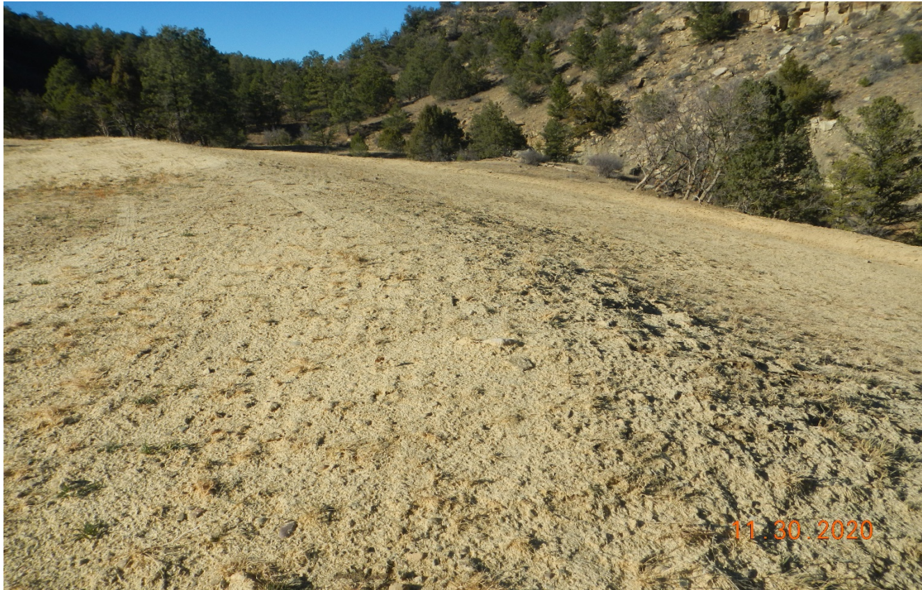
Photo 2. The fill slope has been seeded and stabilized.
