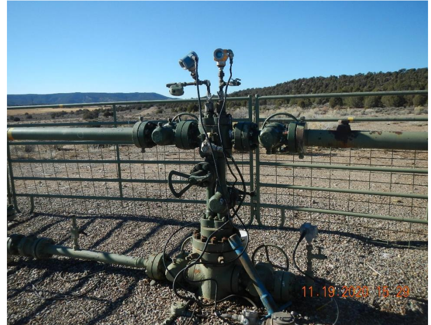
Simms #1A well head. Dual completion.
