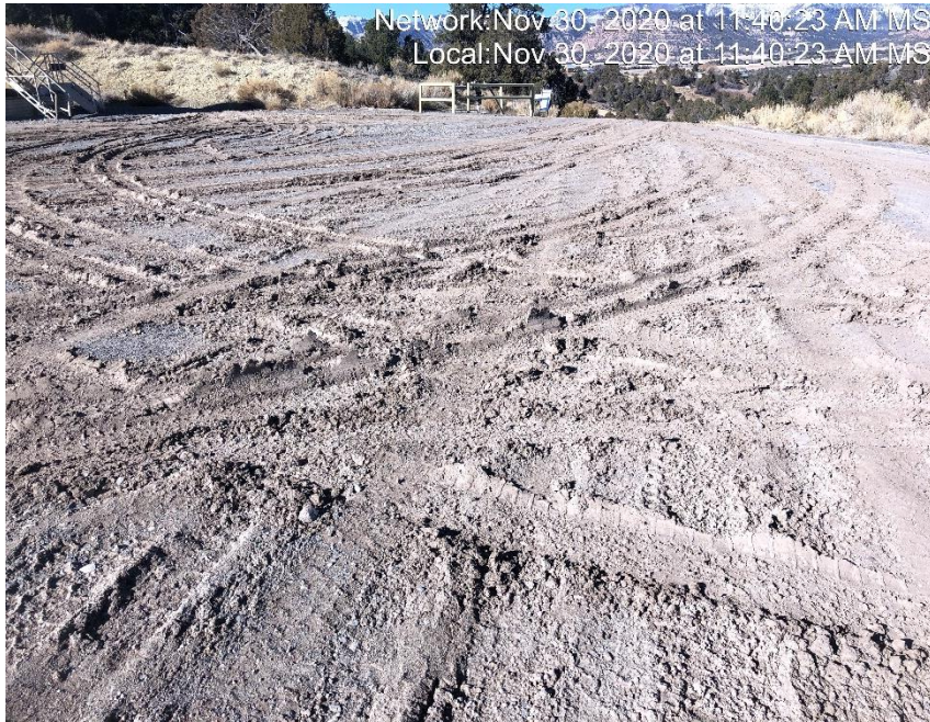
Photo #2340 Sediment is being transported off of location due to tracking.
