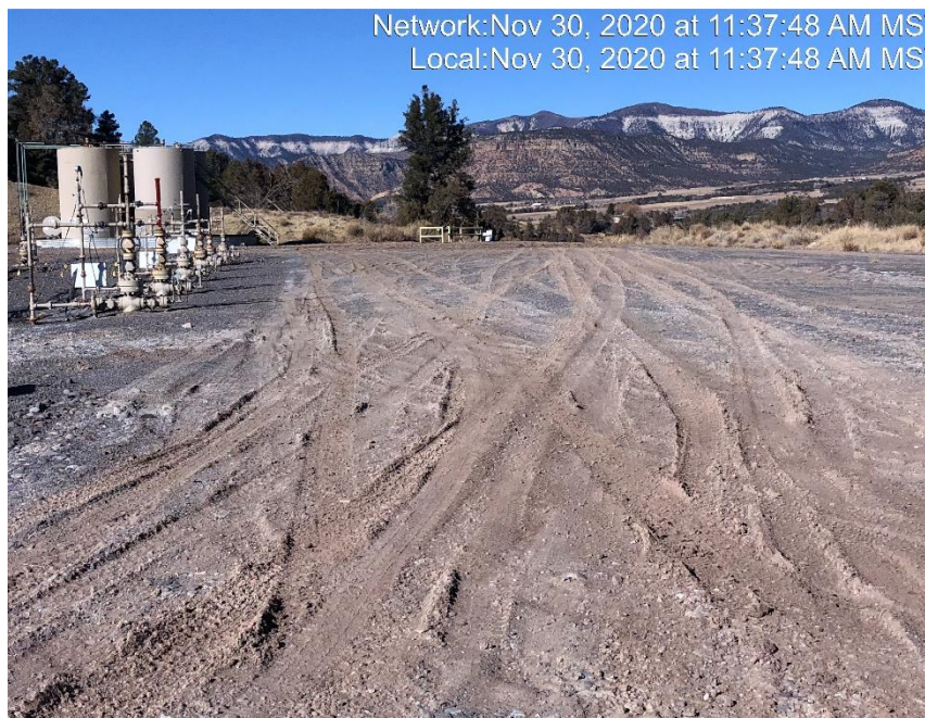
Photo #2338 Sediment is being transported off of location due to tracking.
