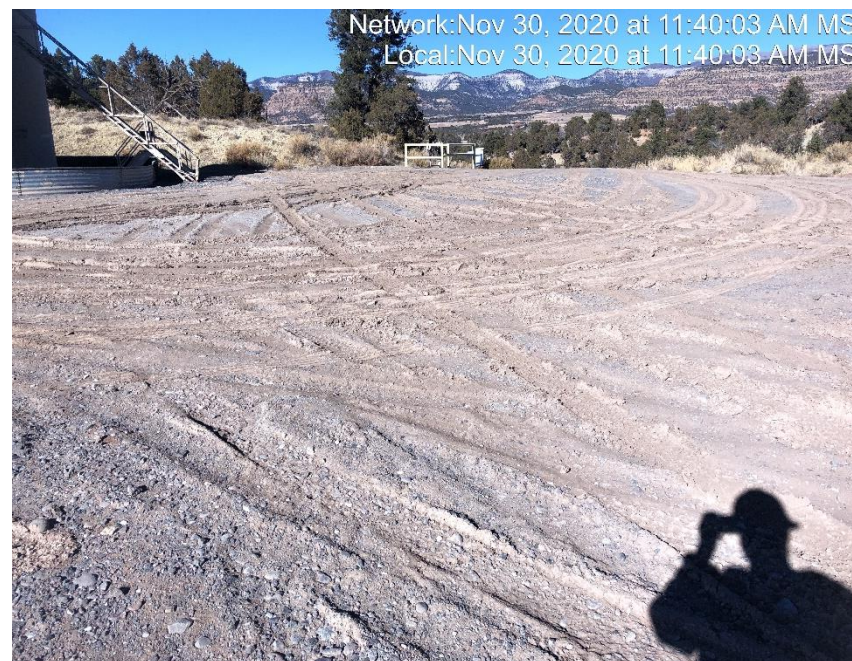
Photo #2339 Sediment is being transported off of location due to tracking.
