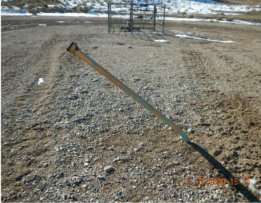
Open ended unused 2" flow line riser in front of well.
