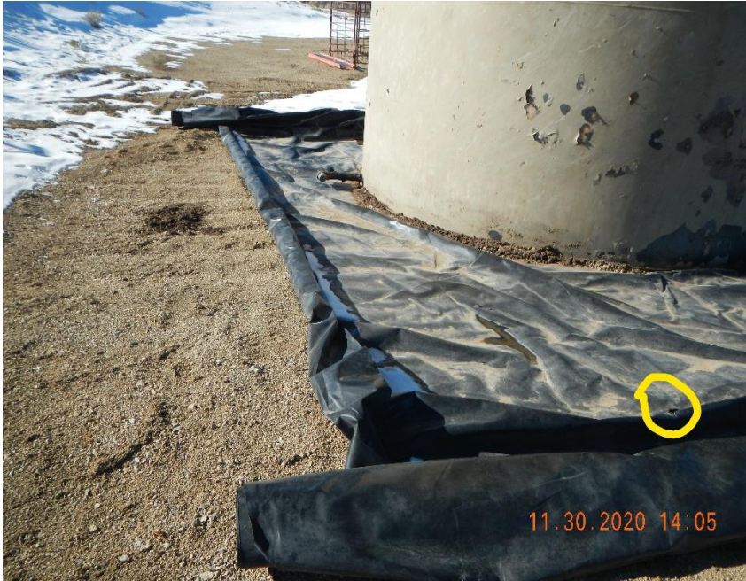
Tear in the plastic liner.
