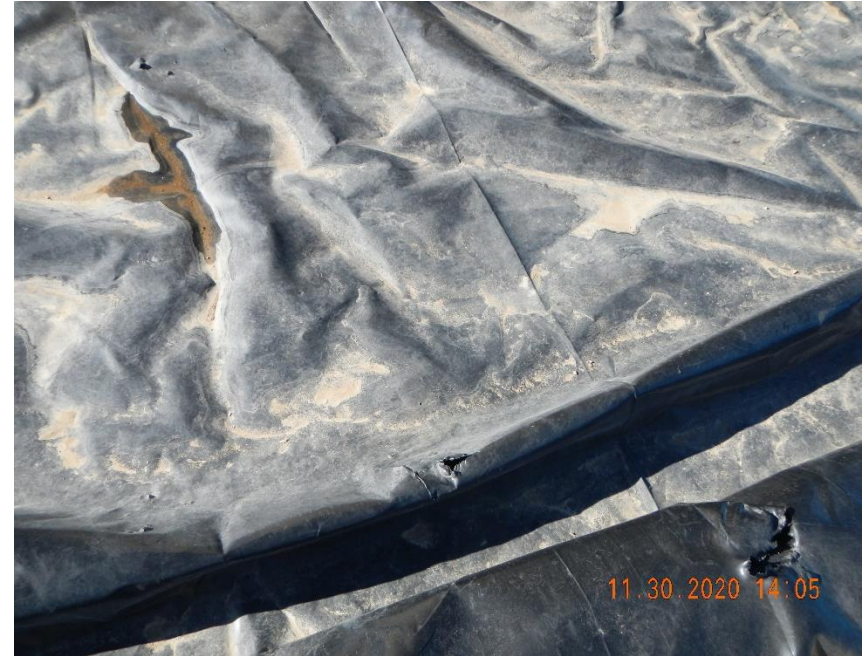
Tear in the plastic liner.
