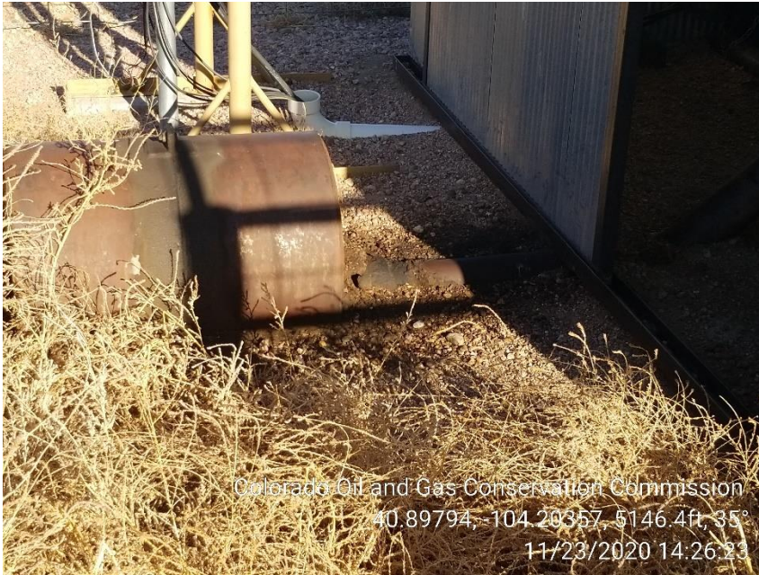
Photo 3 – Stained Soil at Exhaust
