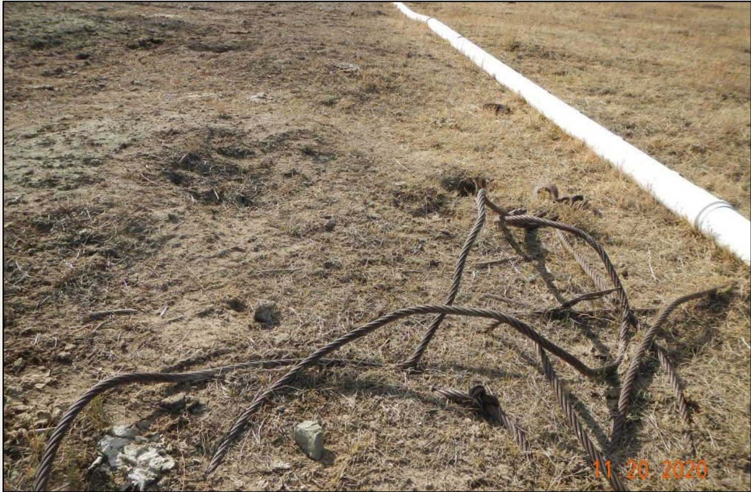
Photo 4. View of cable debris within the western project area.
