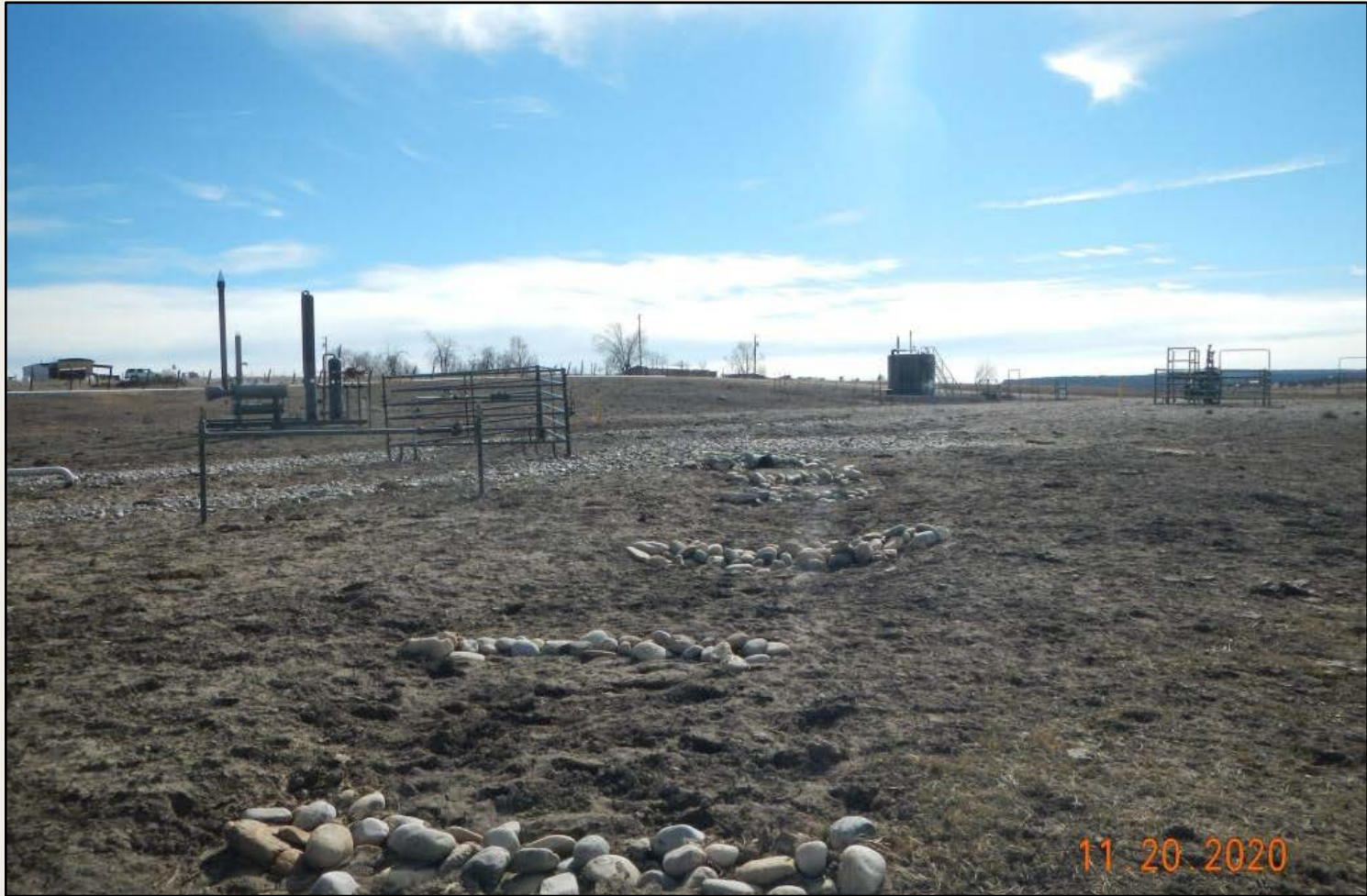
Photo 3. View of cobble checks placed within the project area. Checks are filling with sediment and will soon require maintenance.
