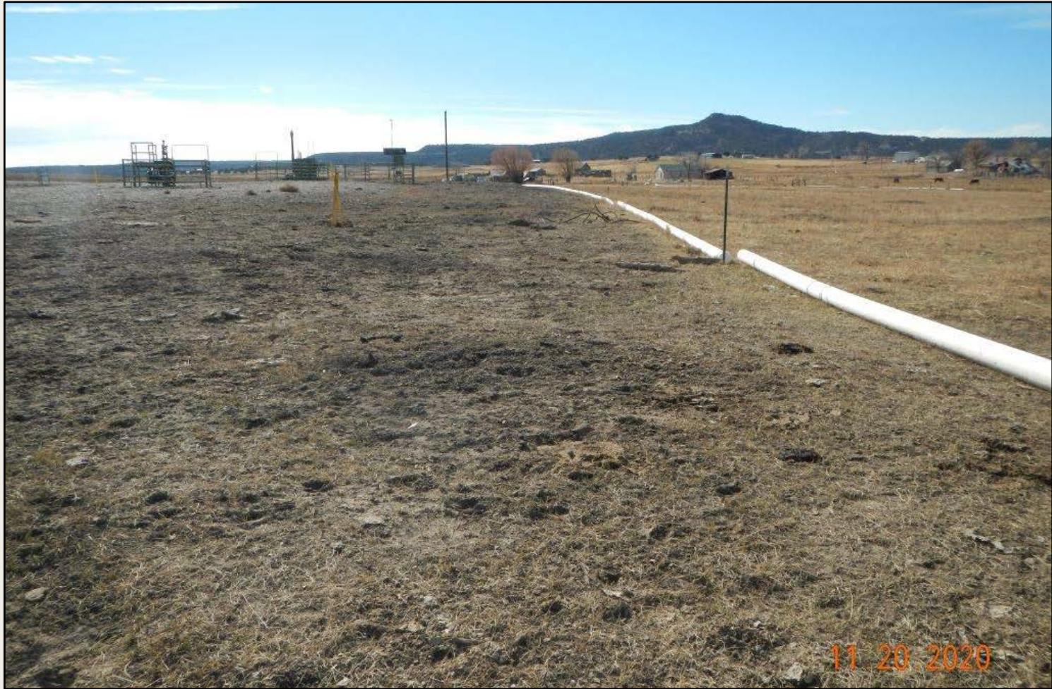
Photo 2. View of the western fill slope from the northwestern corner facing southward. Area is upslope from irrigation alignment, with grasses established in a more sparse and grazed condition than down slope, below irrigation.
