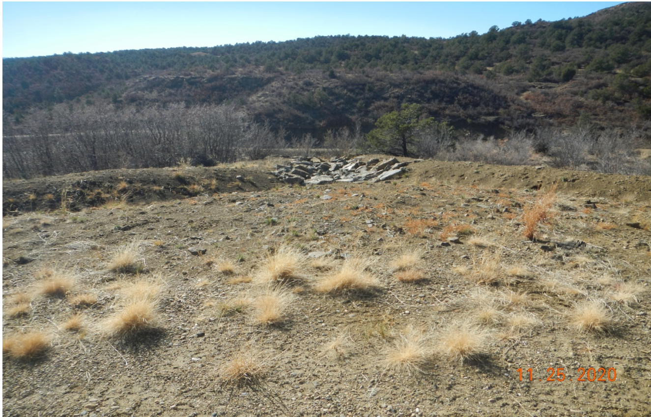
Photo 3. There are berms directed toward this rock rip/rap outlet along the fill slope.
