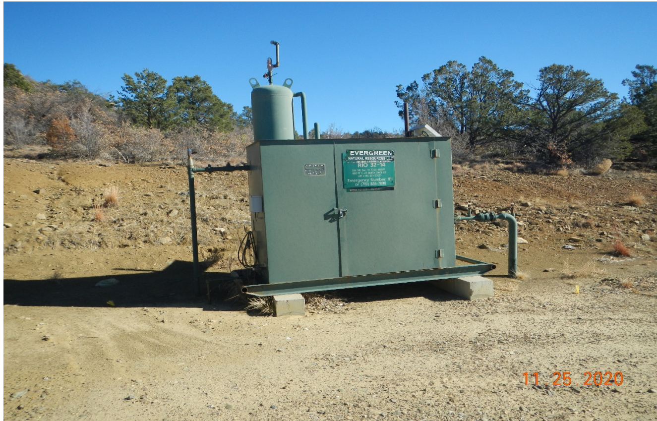
Photo 2. Well sign posted at meter shed.
