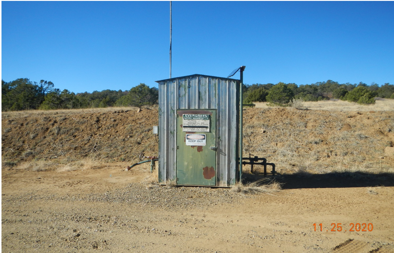
Photo 2. Well sign posted at meter shed.
