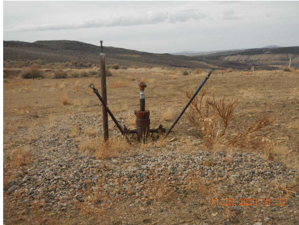
Photo 1. Photo of location taken facing west. No OWP information. No bradenhead access apparent.
