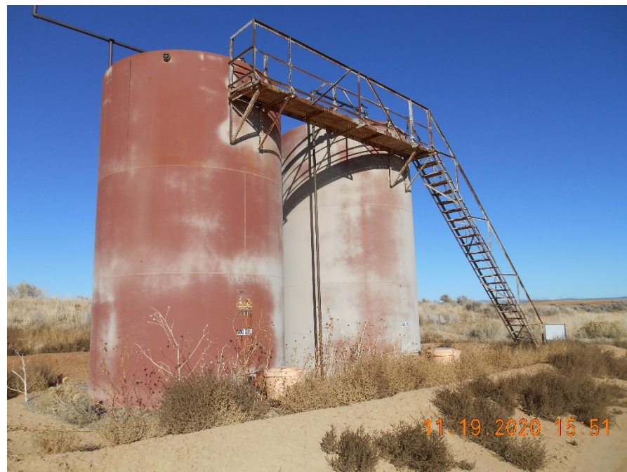
Tank Battery with earth berms.
