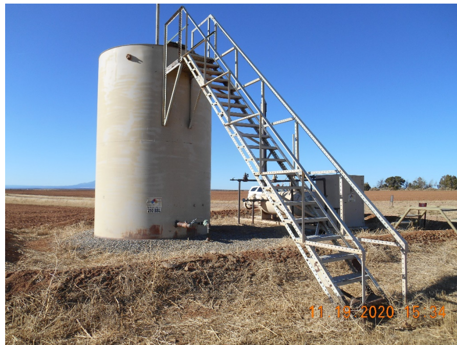
Tank Battery with earth berms.
