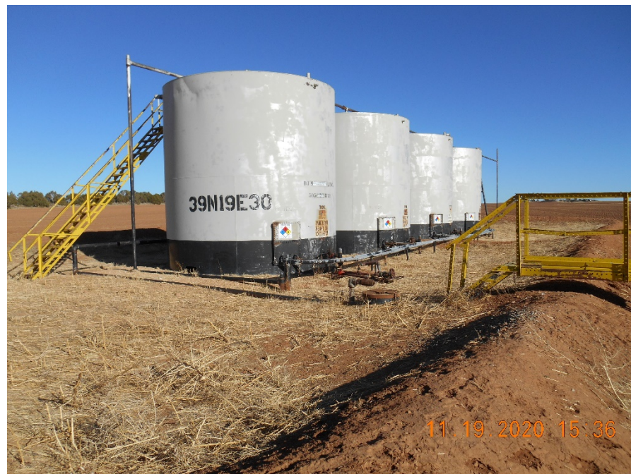
Tank Battery with earth berms.
