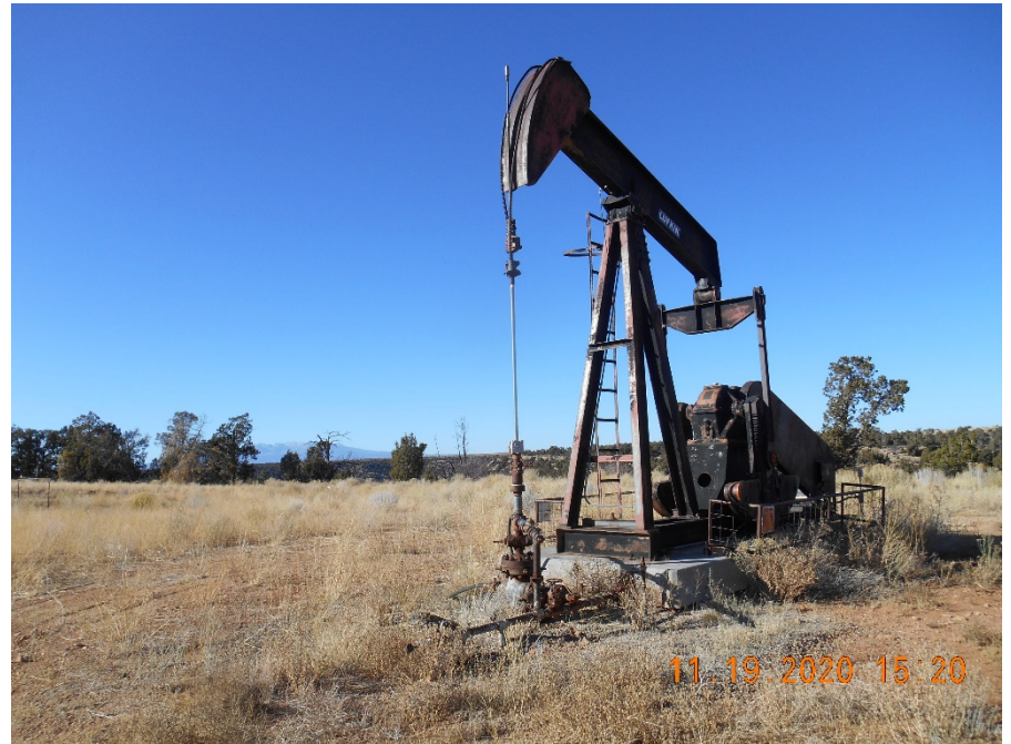
Wellhead with Pump Jack
