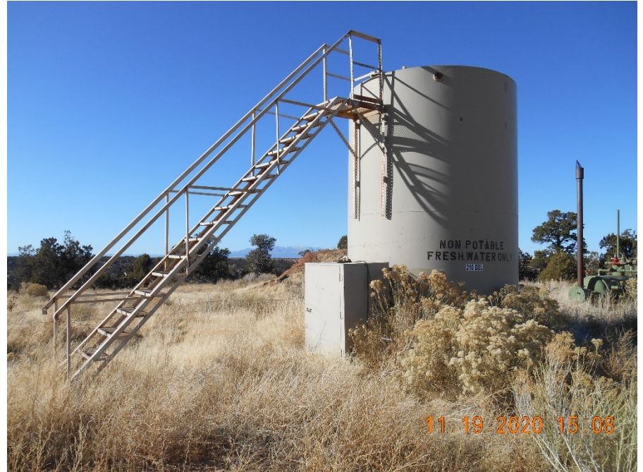
Tank Battery (Fresh Water)
