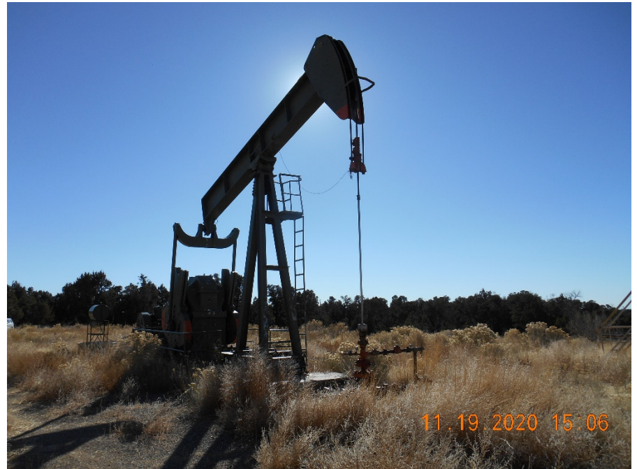
Wellhead with Pump Jack
