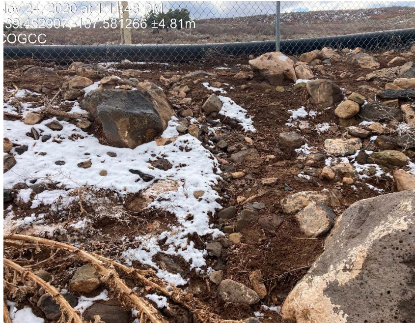
Lack of stabilization/erosion looking west at pad
