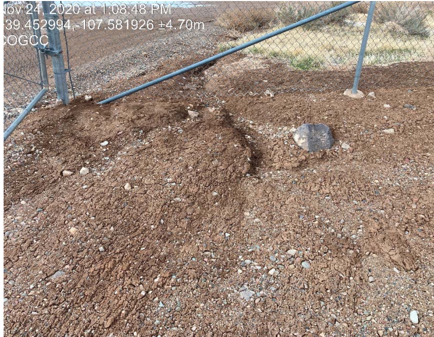
Lack of stabilization/erosion looking north at entrance
