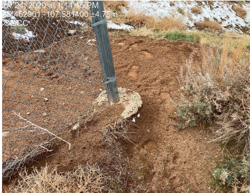
Lack of stabilization/erosion North East corner
