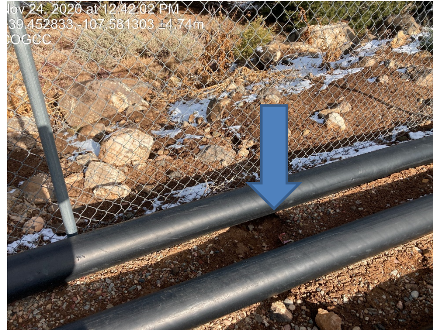
Lack of stabilization/erosion looking East from on the pad
