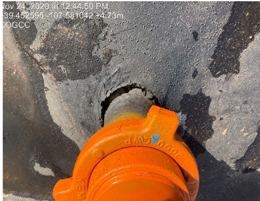
Tank battery containment liner around pipe coming through bottom
