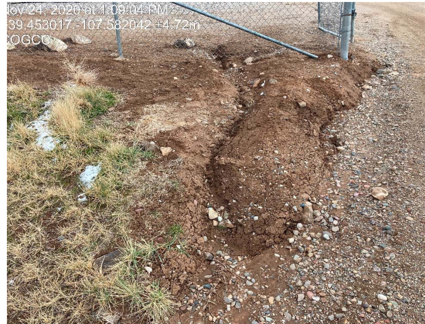
Lack of stabilization/erosion looking south at entrance
