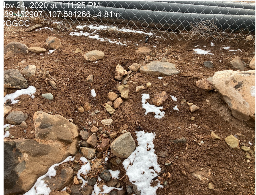
Lack of stabilization/erosion looking west at pad
