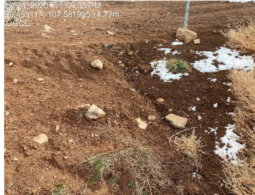
Lack of stabilization/erosion North East corner
