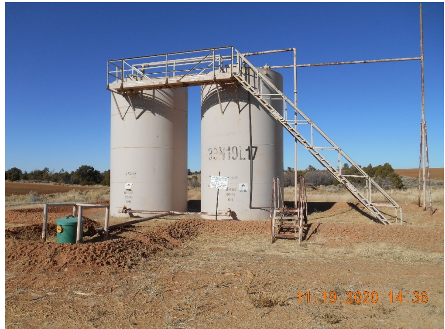
Tank Battery with earth berms.
