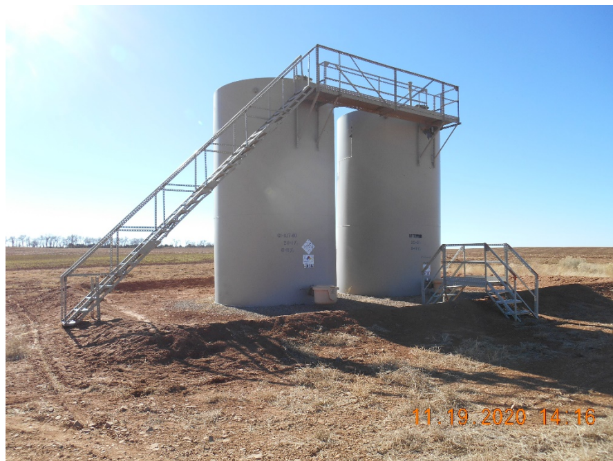
Tank battery with earth berms.
