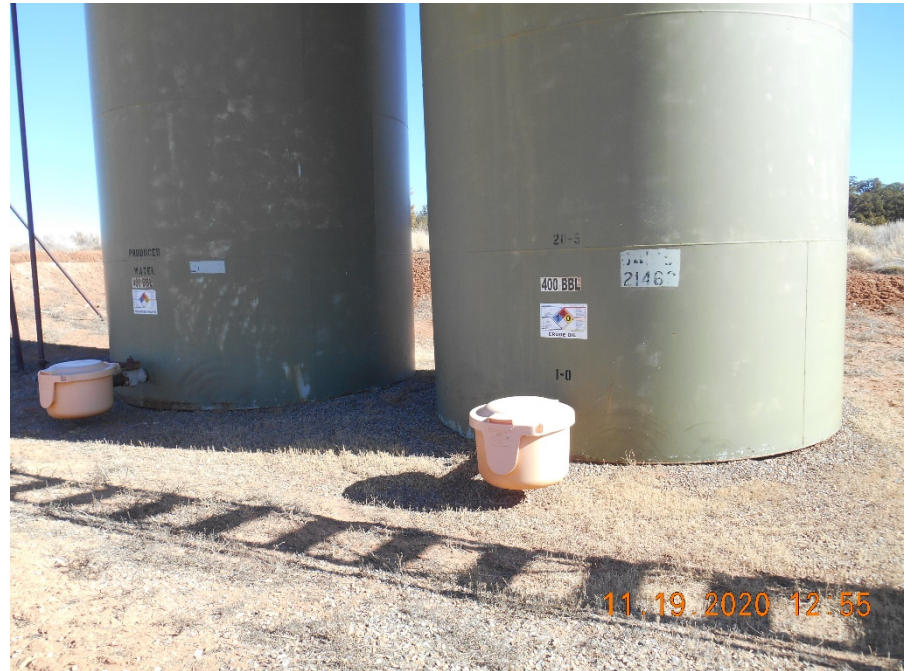
Tank Battery with improper labeling.
