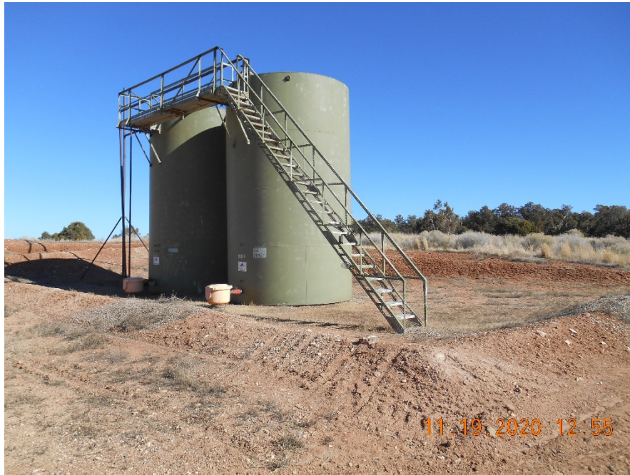
Tank Battery with earth berms. Weeds removed.
