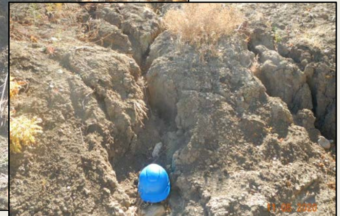
Photo 3. View of eroding area shown in Photo 2, facing up-slope. Erosional channels up to 1 foot wide and 2 feet deep in this area where stormwater flows off of the northwestern well pad. Blue hardhat placed in photo inset for scale.
