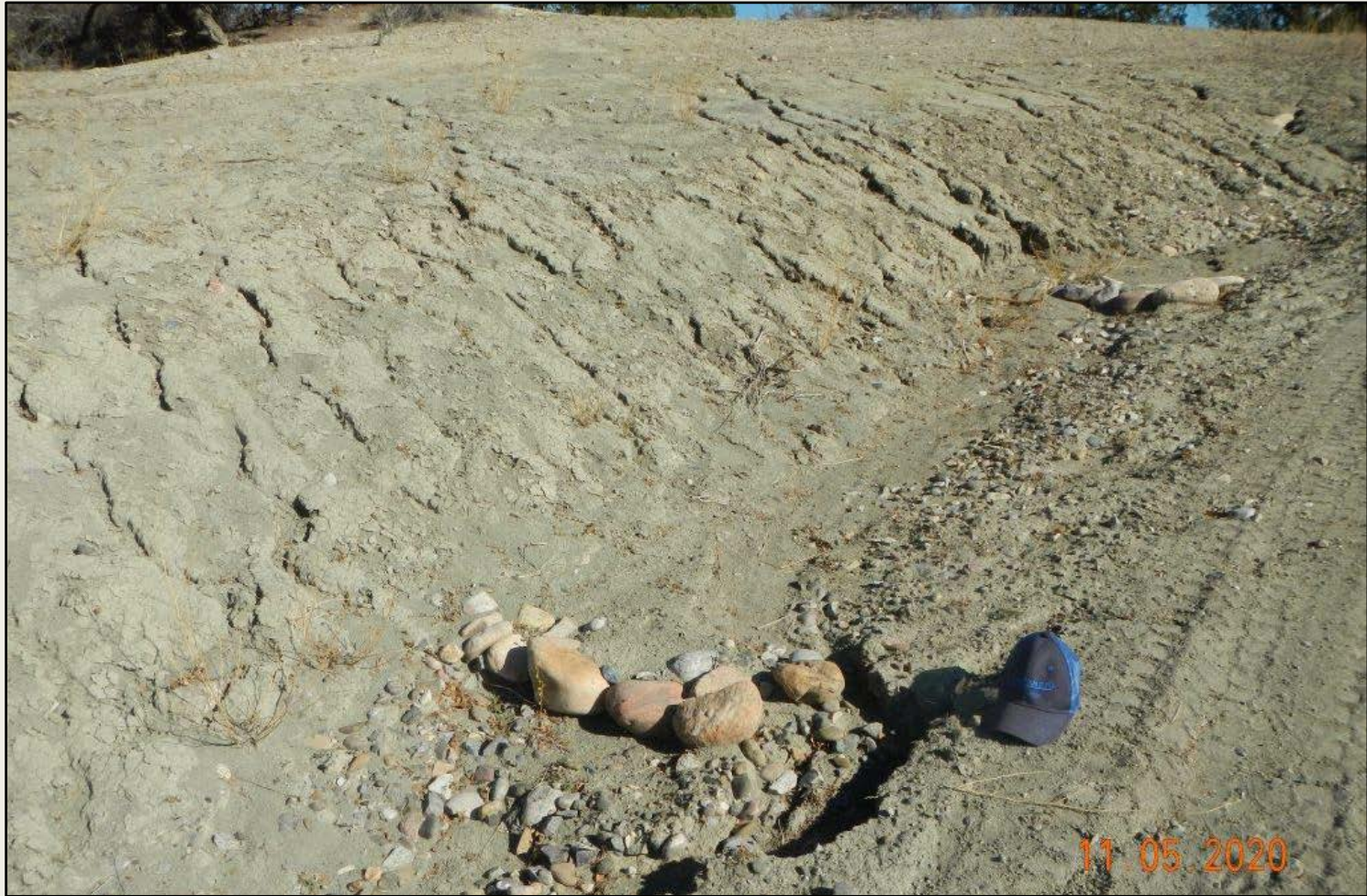
Photo 11. View of erosional rilling along the access road, and sediment filled cobble BMPs along the access. Slope is not stabilized, these BMPs are not adequate here.
