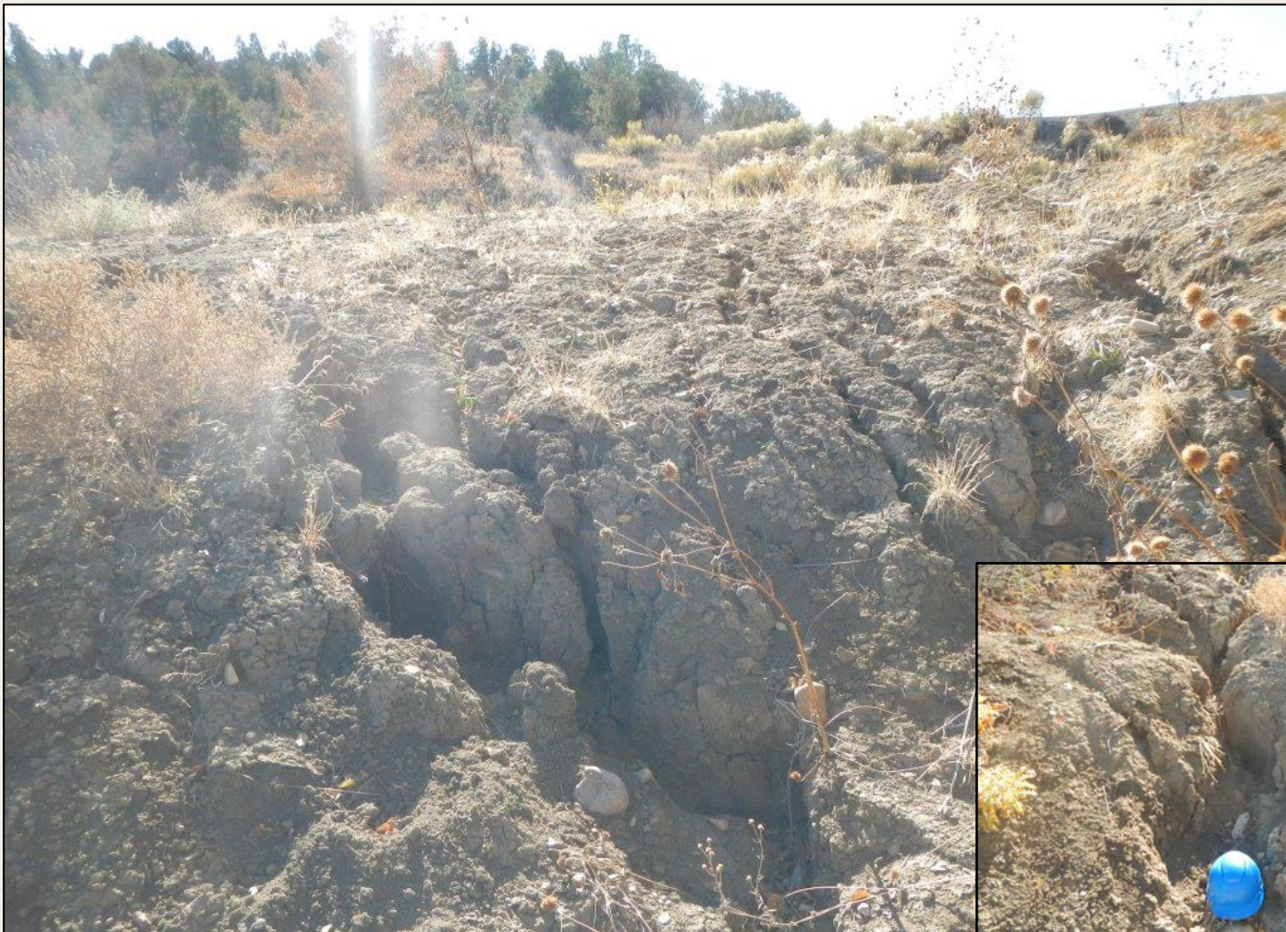
Photo 3. View of eroding area shown in Photo 2, facing up-slope. Erosional channels up to 1 foot wide and 2 feet deep in this area where stormwater flows off of the northwestern well pad. Blue hardhat placed in photo inset for scale.
