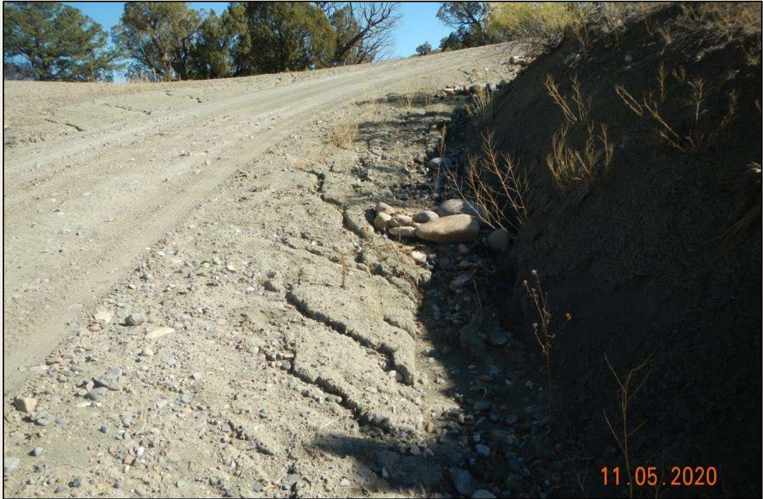
Photo 13. View of another area along the access road where shoulders are not stabilized with evident rilling and cobble BMPs that are inundated with sediment.
