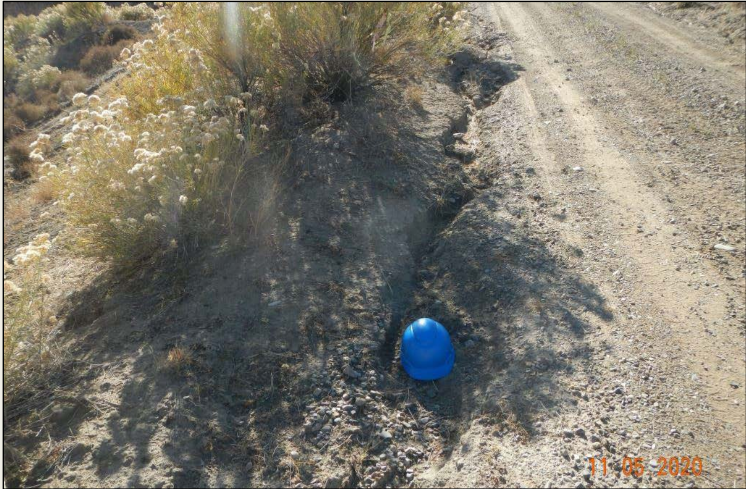
Photo 3. View of erosional channeling, approximately 10-12 inches deep, and 12 to 24 inches wide, occurring along the access- near the well pad entrance.
