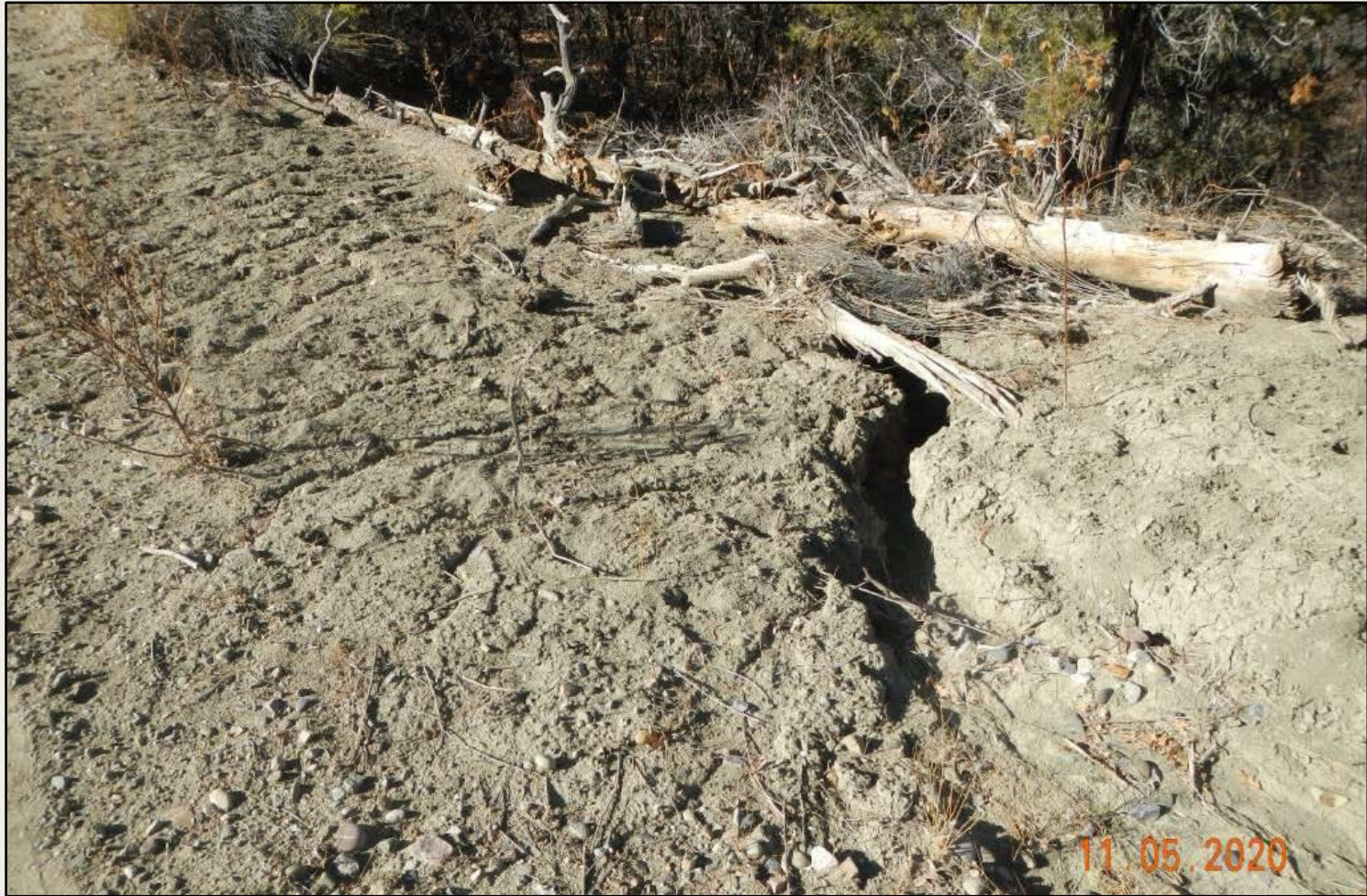
Photo 7. View of erosional rilling and channeling (approximately 1 foot wide and deep) occurring along the access road where erosional channel was repaired in response to a 2019 reclamation inspection.
