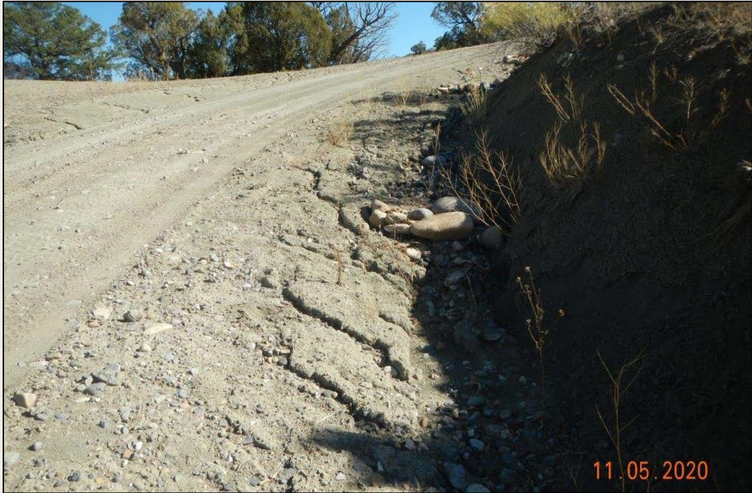
Photo 8. View of another area along the access road where shoulders are not stabilized with evident rilling and cobble BMPs that are inundated with sediment.
