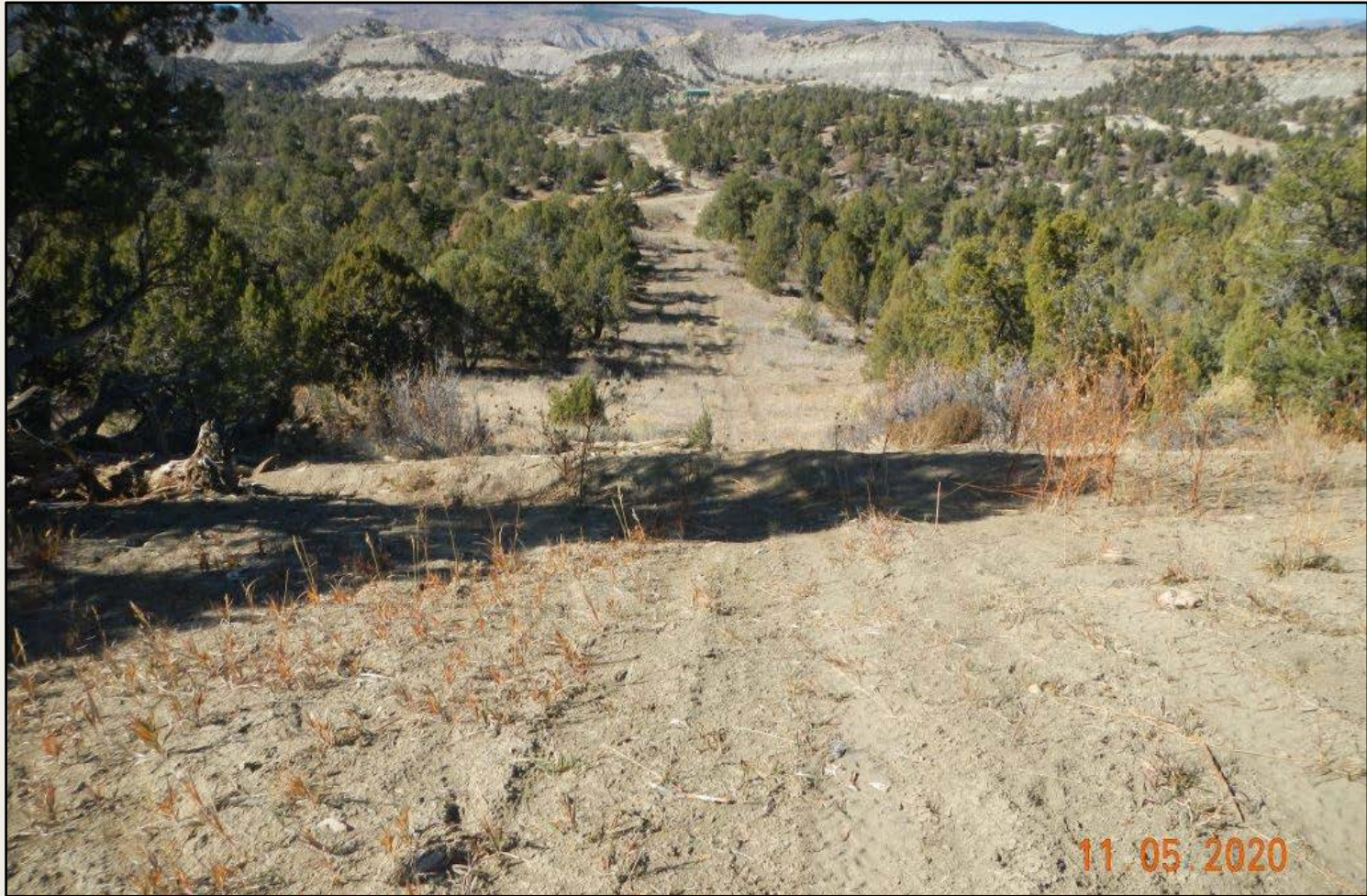
Photo 5. View of pipeline reclamation corridor. Vehicle tracking is damaging vegetation and threatening stabilization.
