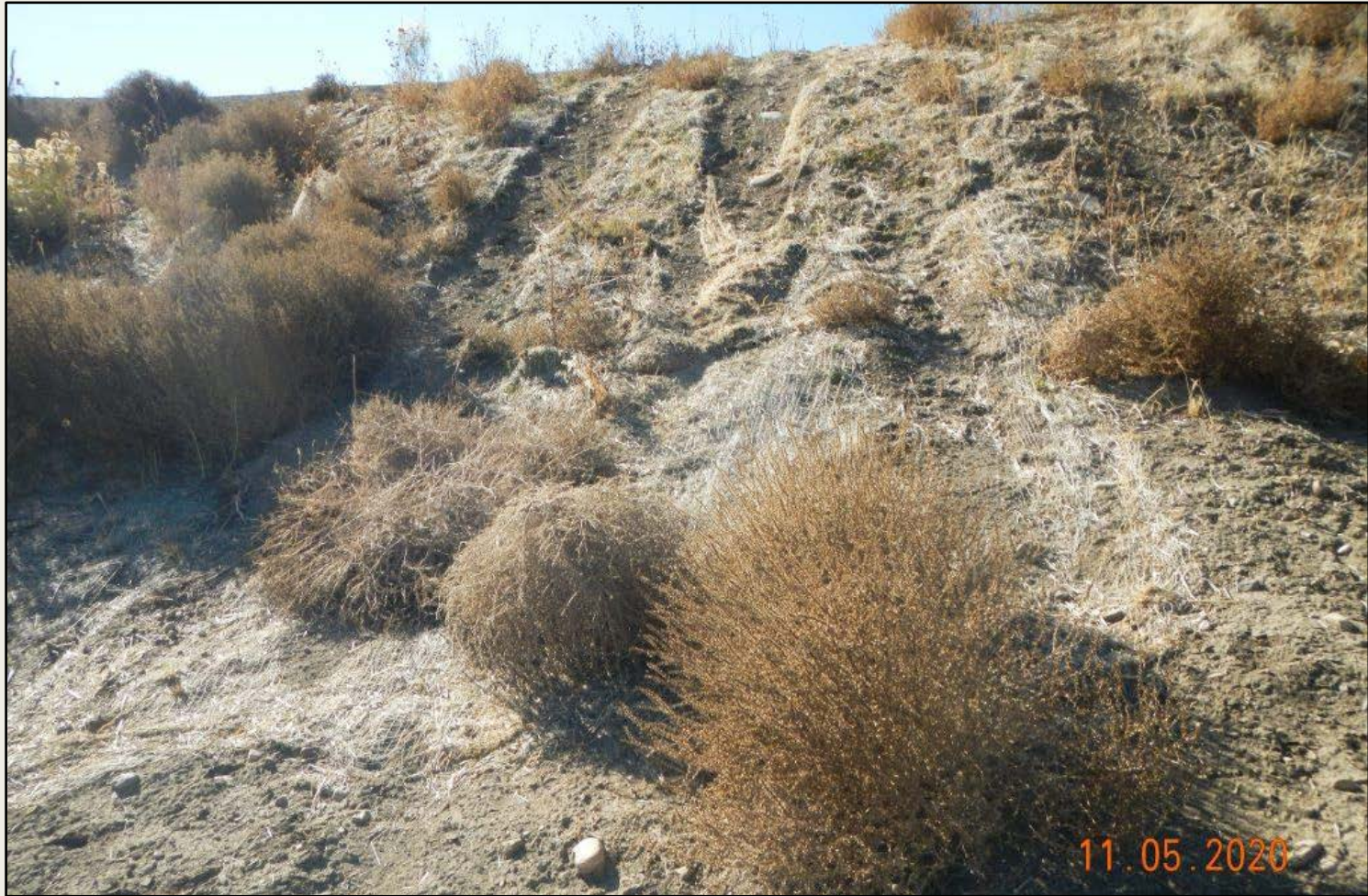
Photo 4. View of tracking damage on straw blanket in the northeastern fill slope. Russian thistle debris is present.
