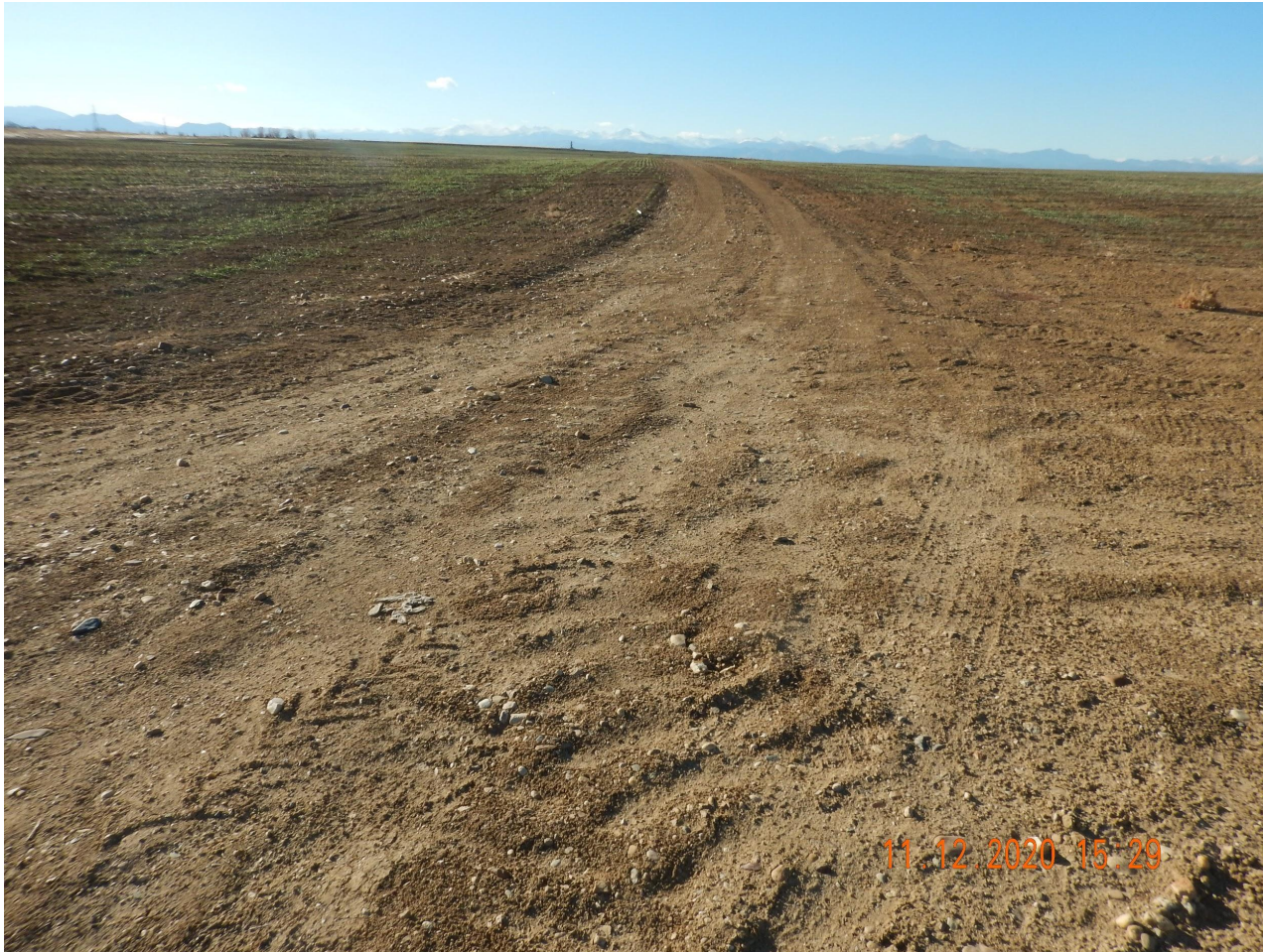
Photo 2. Photo taken from the eastern access road, facing West. Photo illustrates the Operator has failed to perform final reclamation activities for the access road.
