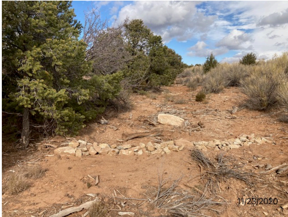
SC-9 Well Location: Storm water controls installed along the western project boundary.
