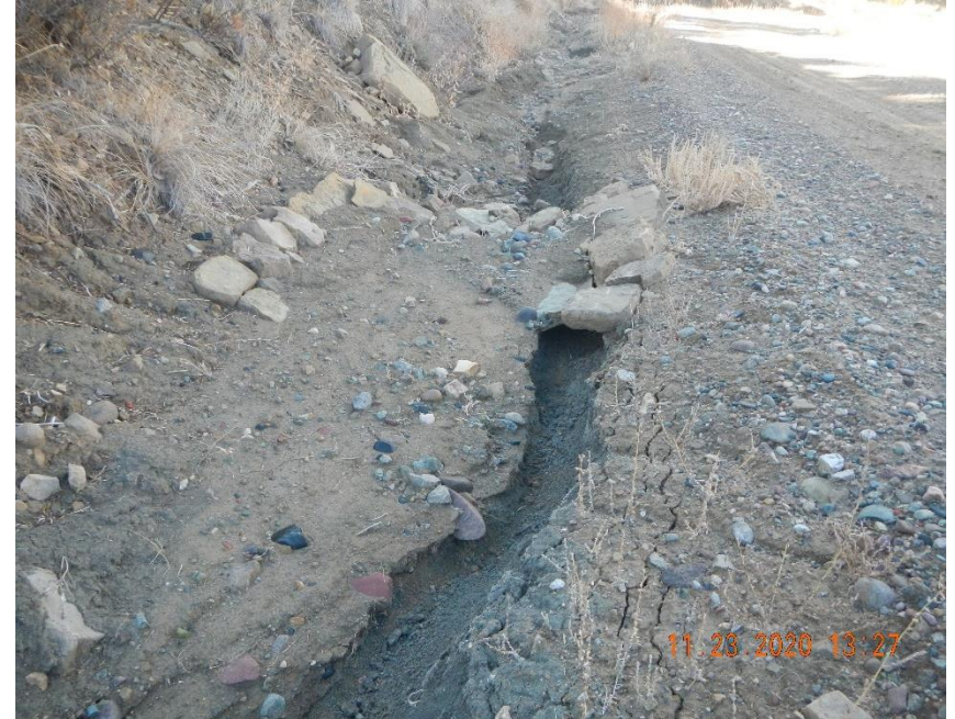
Channeling under rip rap in ditch.
