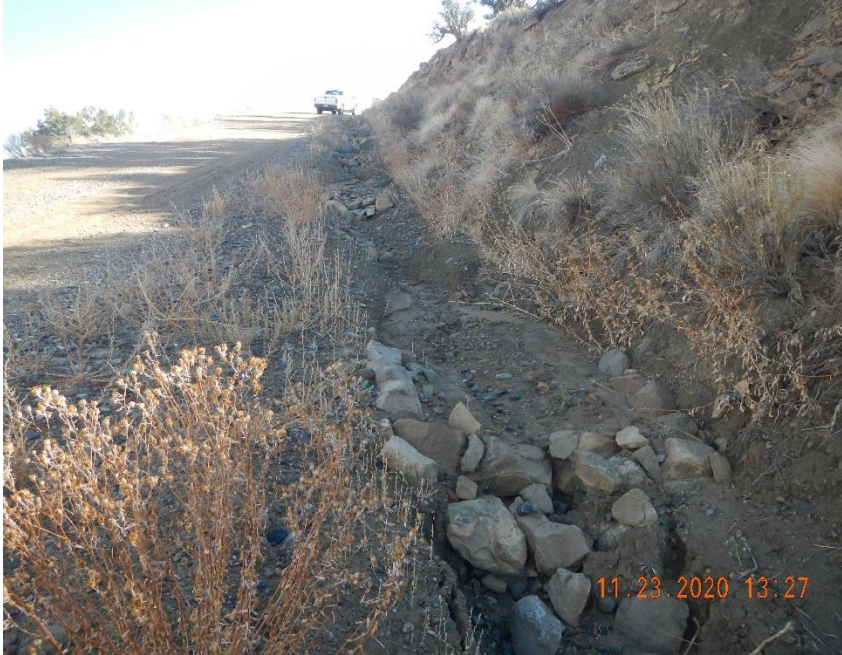
Road ditch needs maintained. Coordinates 39.47075 W108.10118
