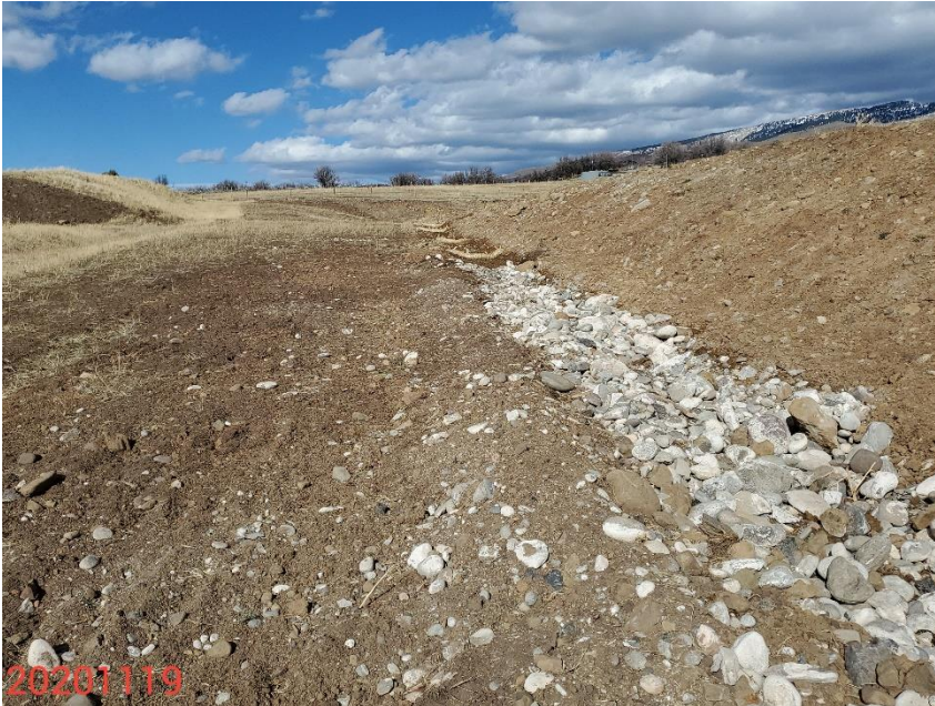
Photo 3: Photo taken from the stormwater ditch on the west end of the Location, facing north. Photo shows ditch BMP has not been constructed in accordance with good engineering per the sites conditions.
