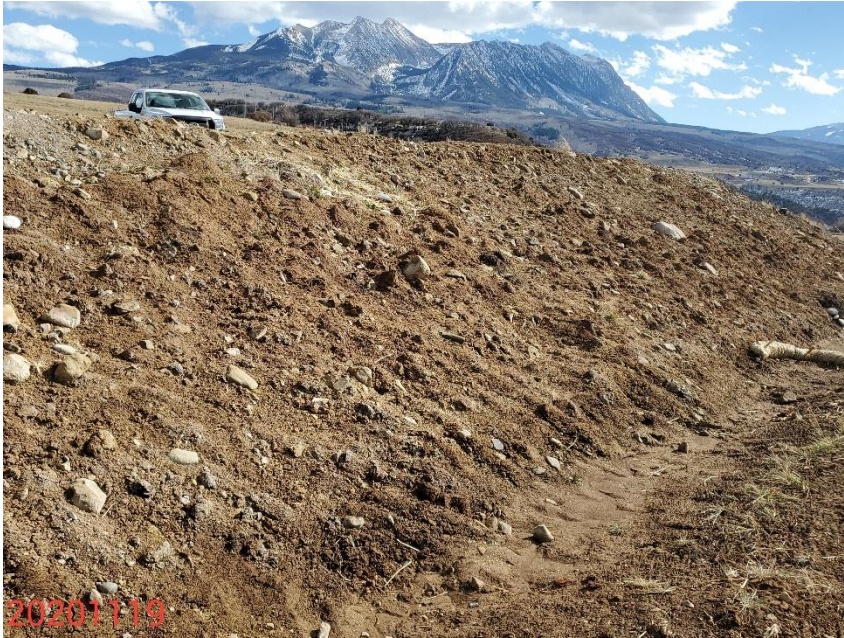
Photo 5: Photo taken from the west end of the Location, facing south east. Photo shows example of slopes on the Location where stabilization BMPs remain missing or insufficient.
