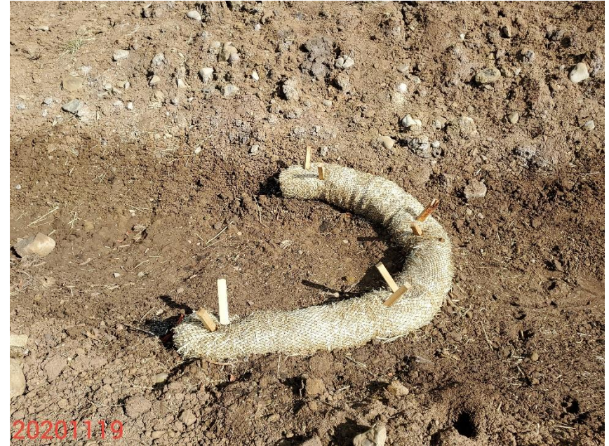
Photo 4: Photo taken from the stormwater ditch. Photo shows straw wattle as a velocity check in the ditch.
