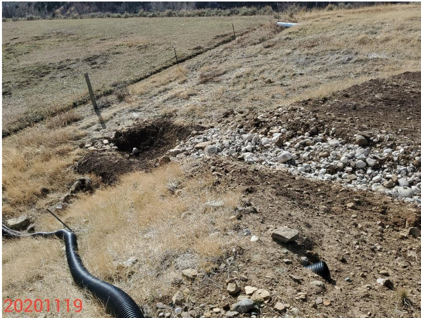
Photo 1: Photo taken from the stormwater ditch on the west end of the Location. Operator has installed a sediment trap. BMP insufficient in size for the site's conditions and have not been installed in accordance with good engineering practices.
