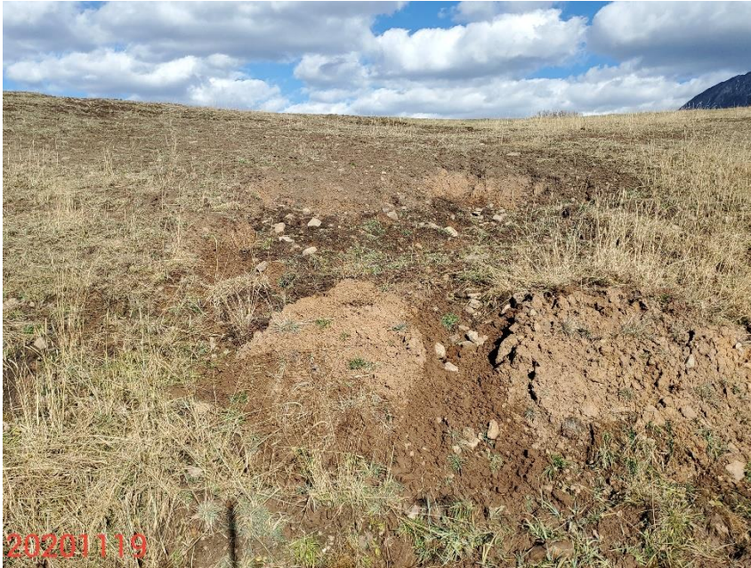
Photo 7: Photo taken from the slopes on the north end of the Location, facing north. Photo shows erosion degradation on the northern cut slope. BMPs remain missing or insufficient to stabilize and protect slopes.
