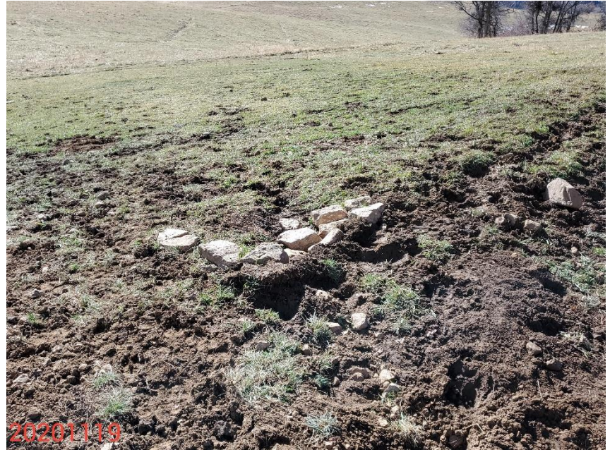
Photo 12: Continued from photo 11. Photo shows outlet at ditch. BMP insufficient as an appropriate outlet to allow for sediment laden-free stormwater discharge.
