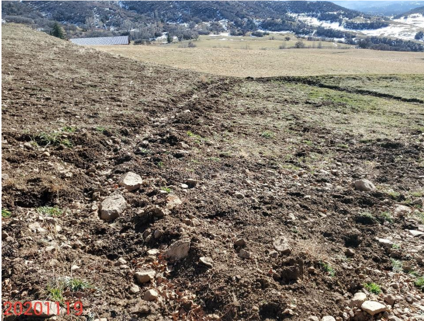
Photo 11: Photo taken from the northwestern end of the Location, facing south. Photo shows ditch BMPs. Photo shows ditch has not been constructed in accordance with good engineering practices.
