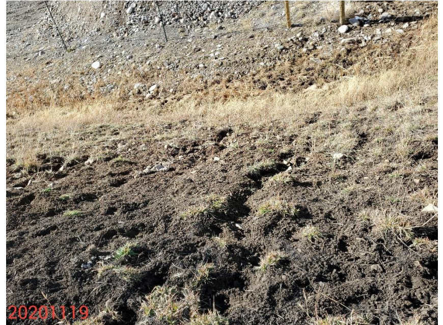
Photo 4: Photo taken from the cut slopes on the northeast corner of the Location. Photo shows BMPs remain missing or insufficient to stabilize and protect slopes.
