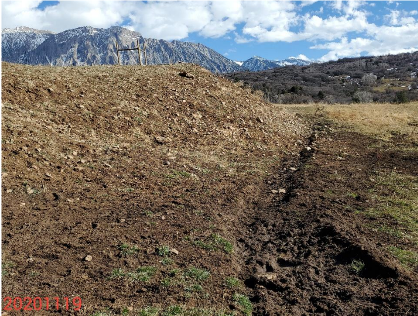
Photo 15: Photo taken from the southwest end of the Location, facing east. Photo shows fill slopes below ditch (photo 13). Photo shows BMPs remain missing or insufficient to protect slopes, and allow for sediment laden-free stormwater discharge from the ditch.
