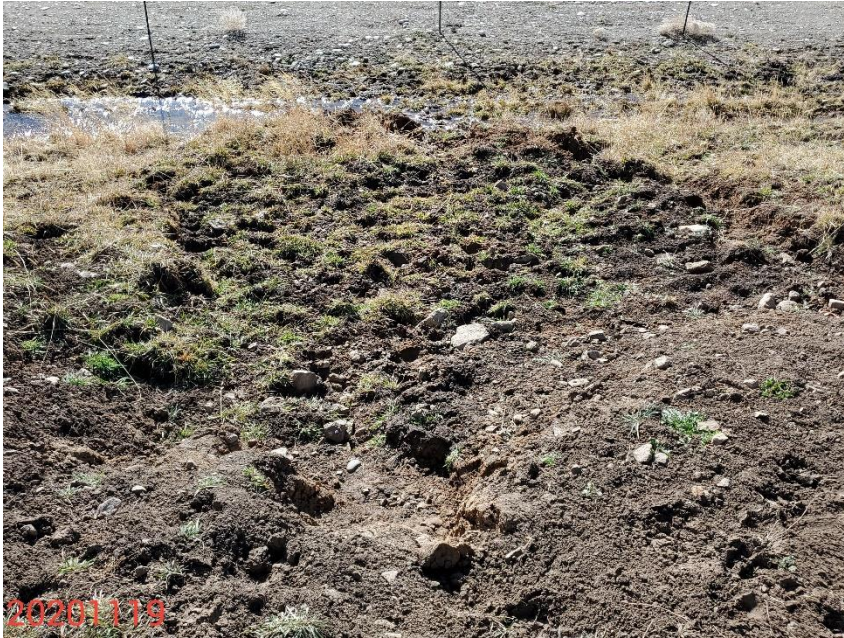
Photo 5: Photo taken from the slopes on the north end of the Location. Photo shows erosion degradation on the northern cut slope. BMPs remain missing or insufficient to stabilize and protect slopes.
