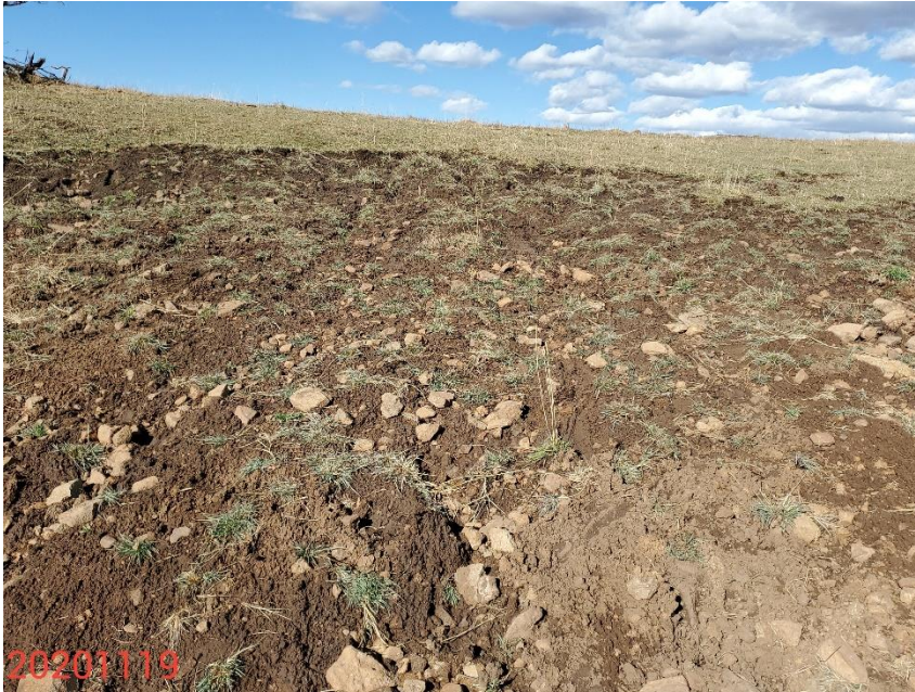
Photo 9: Photo taken from the slopes on the northwestern area of the Location, facing north. Photo shows erosion degradation on the northern cut slope. BMPs remain missing or insufficient to stabilize and protect slopes.
