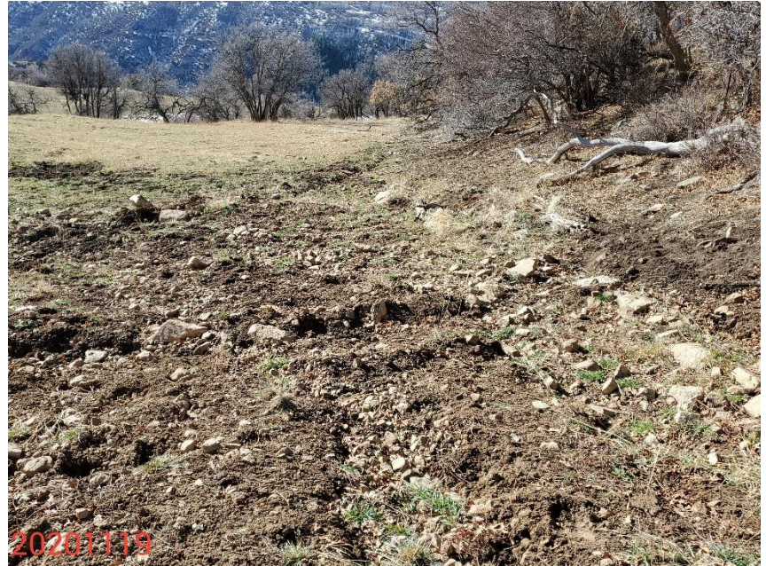
Photo 10: Photo taken from the northwestern end of the Location, facing west. Photo shows ditch BMPs. Photo shows ditch has not been constructed in accordance with good engineering practices. No outlet observed to allow for sediment laden-free stormwater discharge.
