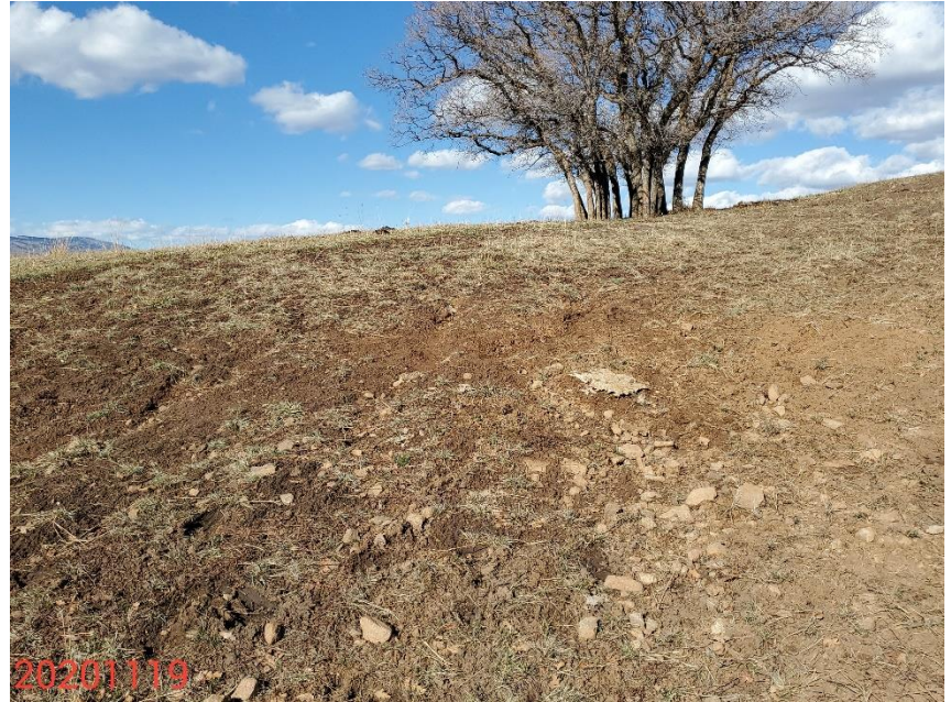
Photo 8: Photo taken from the slopes on the northeastern area of the Location, facing northwest. Photo shows erosion degradation on the northern cut slope. BMPs remain missing or insufficient to stabilize and protect slopes.
