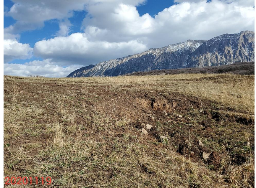
Photo 6: Photo taken from the slopes on the north end of the Location, facing northwest. Photo shows erosion degradation on the northern cut slope. BMPs remain missing or insufficient to stabilize and protect slopes.
