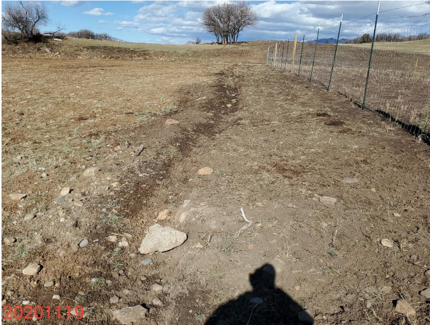
Photo 13: Photo taken from the southwest corner of the Location, facing north. Photo shows perimeter stormwater ditch. Ditch BMP has not been constructed in accordance with good engineering practices; BMP ends on the southwest end of the location and does not have a sufficient outlet to allow for sediment laden-free stormwater discharge.
