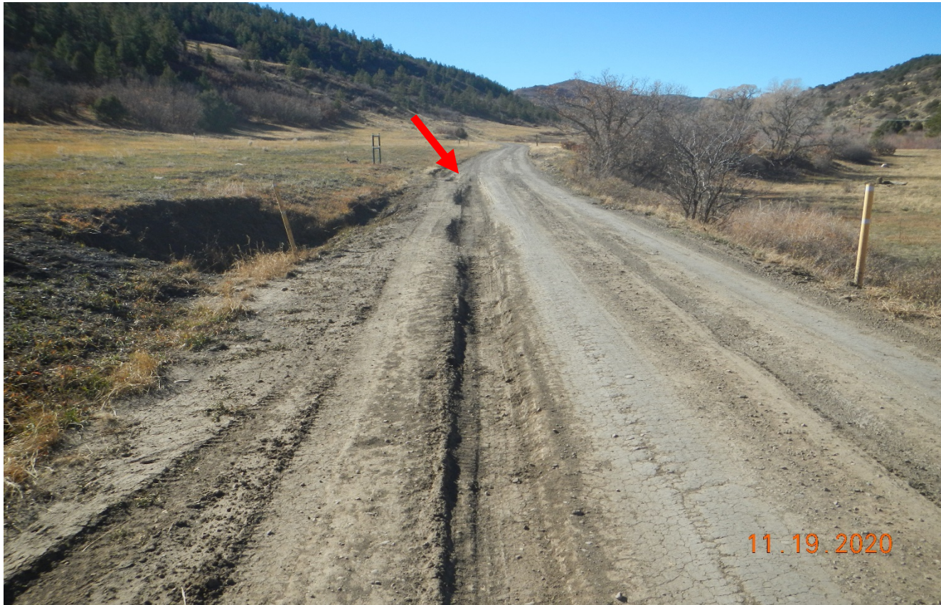
Photo 2. Stormwater is not properly diverted at the red arrow causing stormwater to pool in the vehicle ruts. This area needs to be repaired. (Lat/Long:37.071679,-104.91145)
