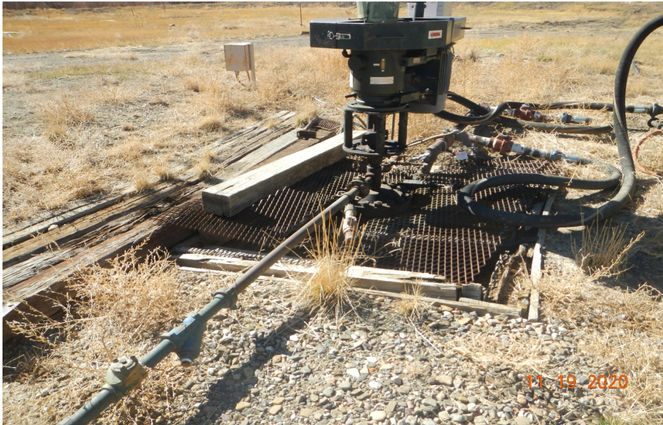
Photo 4. The metal grate at the wellhead is displaced. This area should be maintained and covered to prevent wildlife entry.
