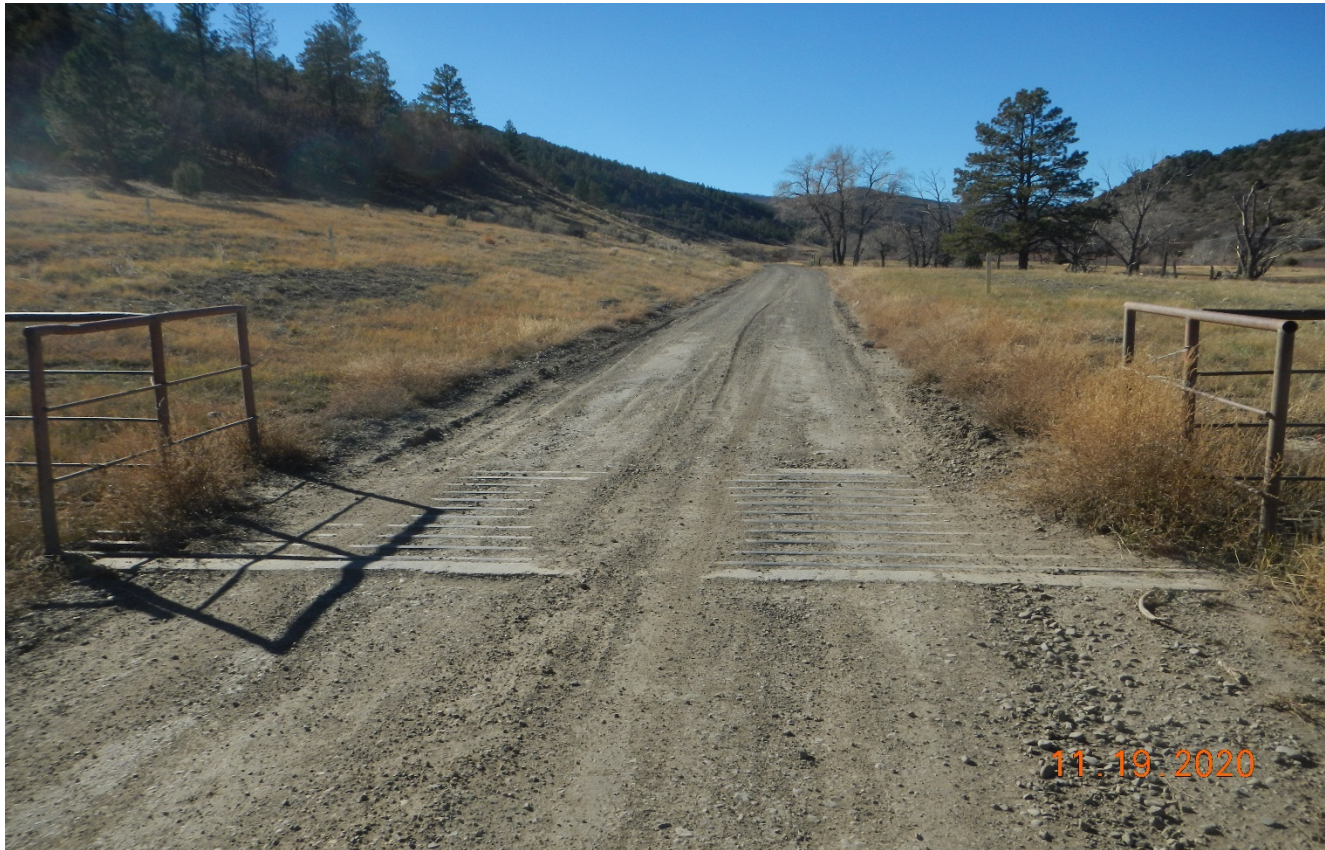
Photo 1. The cattle guard along the main road near the Bingham campground is filled in with sediment. The cattle guard needs to be maintained.
