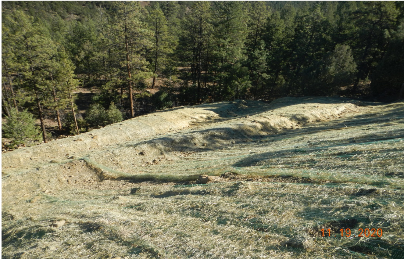
Photo 5. Facing southeast toward the fill slope of the pad.
