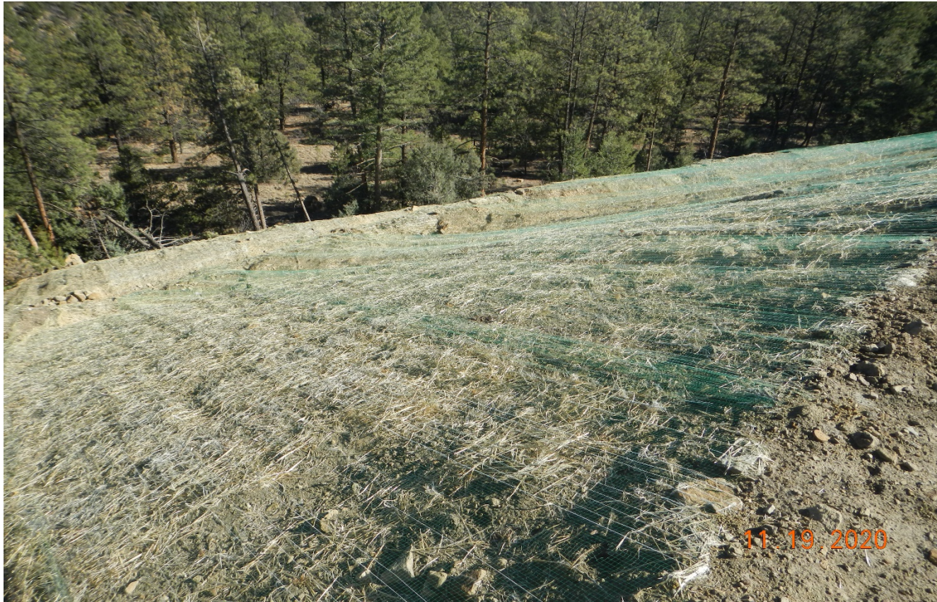
Photo 2. The pad which had sloughed has been recontoured and straw blanket was installed.
