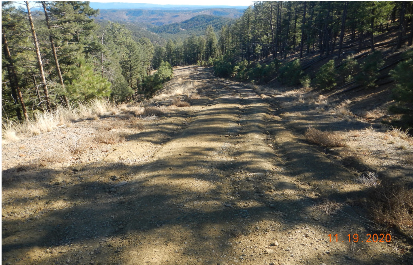
Photo 3. Stormwater is causing erosion down the road.
