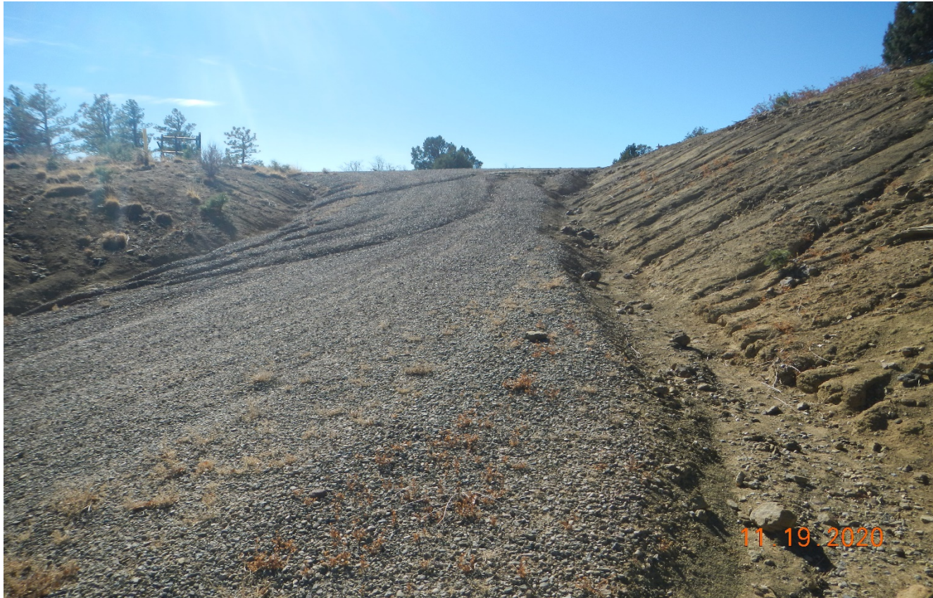
Photo 1. Facing south at the beginning of the access road. There is erosion occurring down the road and the side of the road is not stabilized. Stormwater directed down the road is causing erosion which is shown in the next photo.
