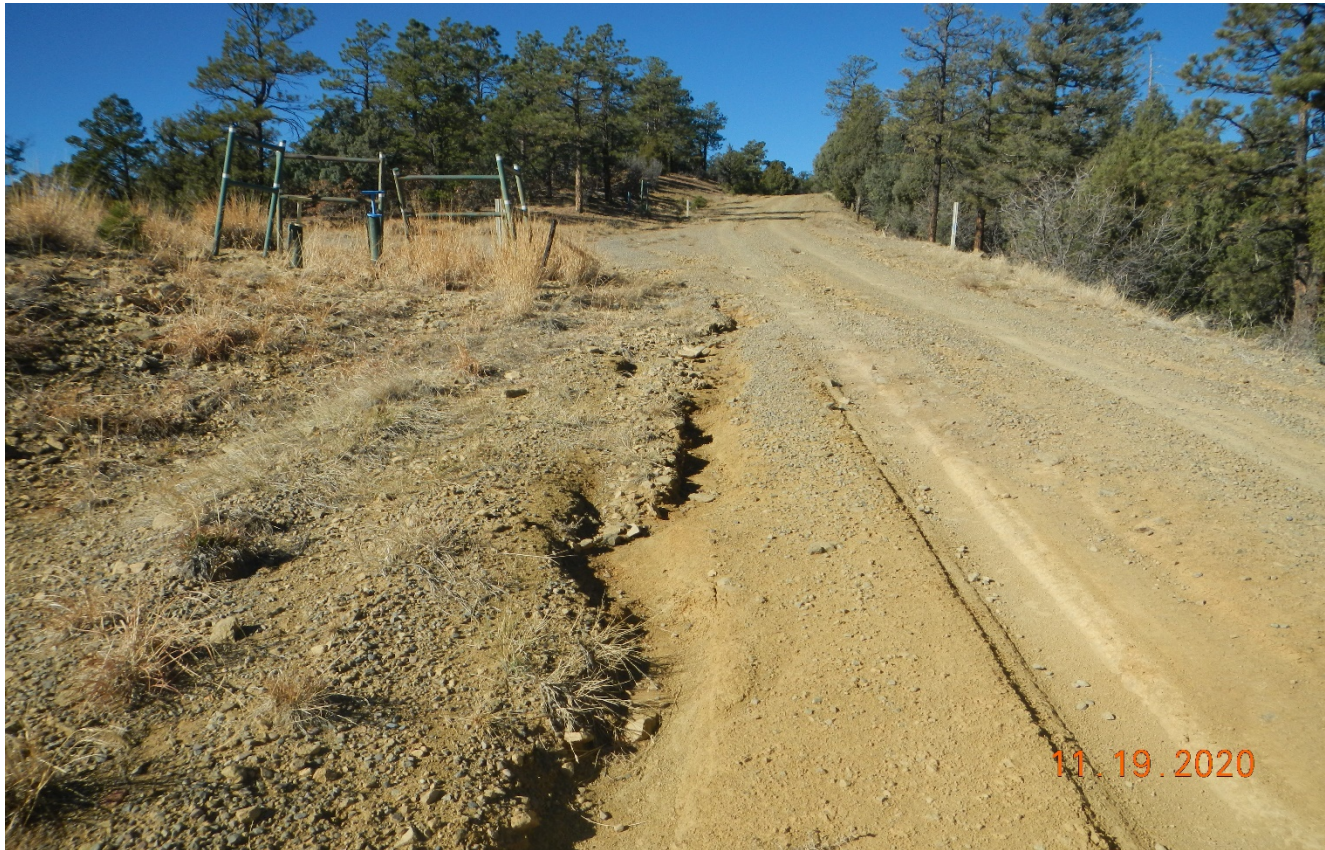
Photo 1. Storm water erosion is occurring down the side of the road. BMP's need to be installed to prevent erosion.
