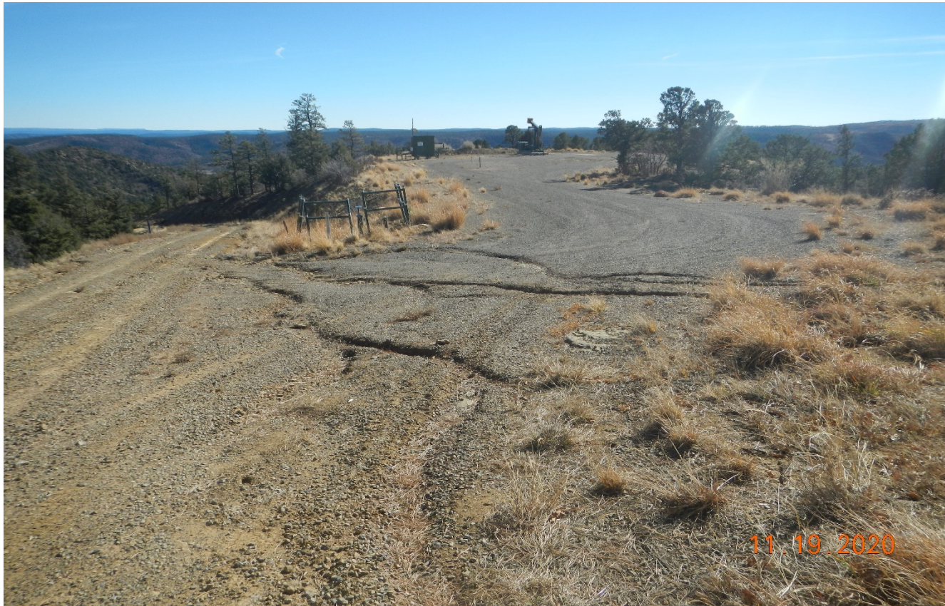
Photo 2. Facing southeast toward the location. Stormwater is causing erosion across and down the road.
