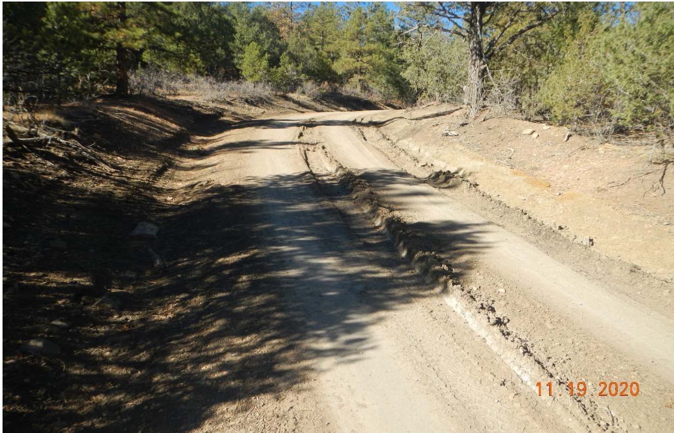
Photo 4. There is vehicle ruts occurring after repairs had been performed. BMP's such as gravel is needed to prevent rutting and road degradation.
