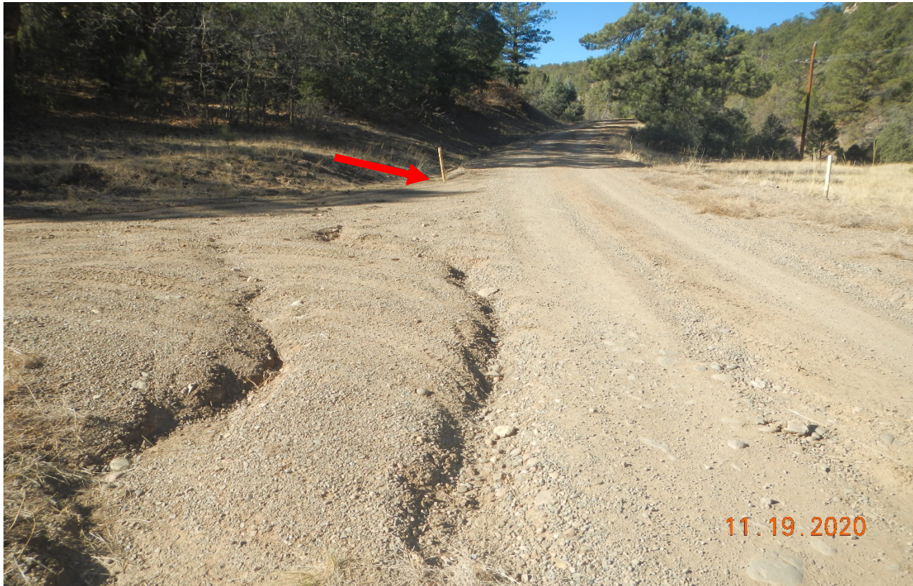
Photo 1. There is a plugged culvert along the main road (red arrow) causing stormwater to flow down the road. Lat/Long:37.09178,-104.93688. Corrective action was not completed.
