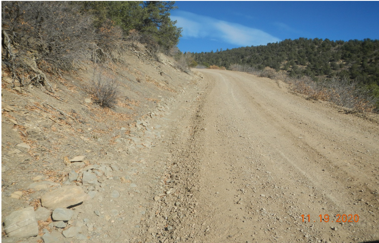
Photo 3. There is a long stretch of road with no BMP's to prevent erosion which was previously observed. Rock along the side could be used for check dams to slow stormwater velocity.
