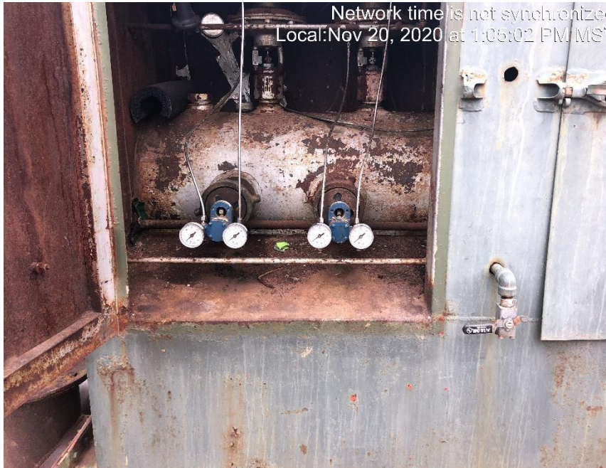
Photo #2300 gas leaking from a dump controller mixer inside the separator.
