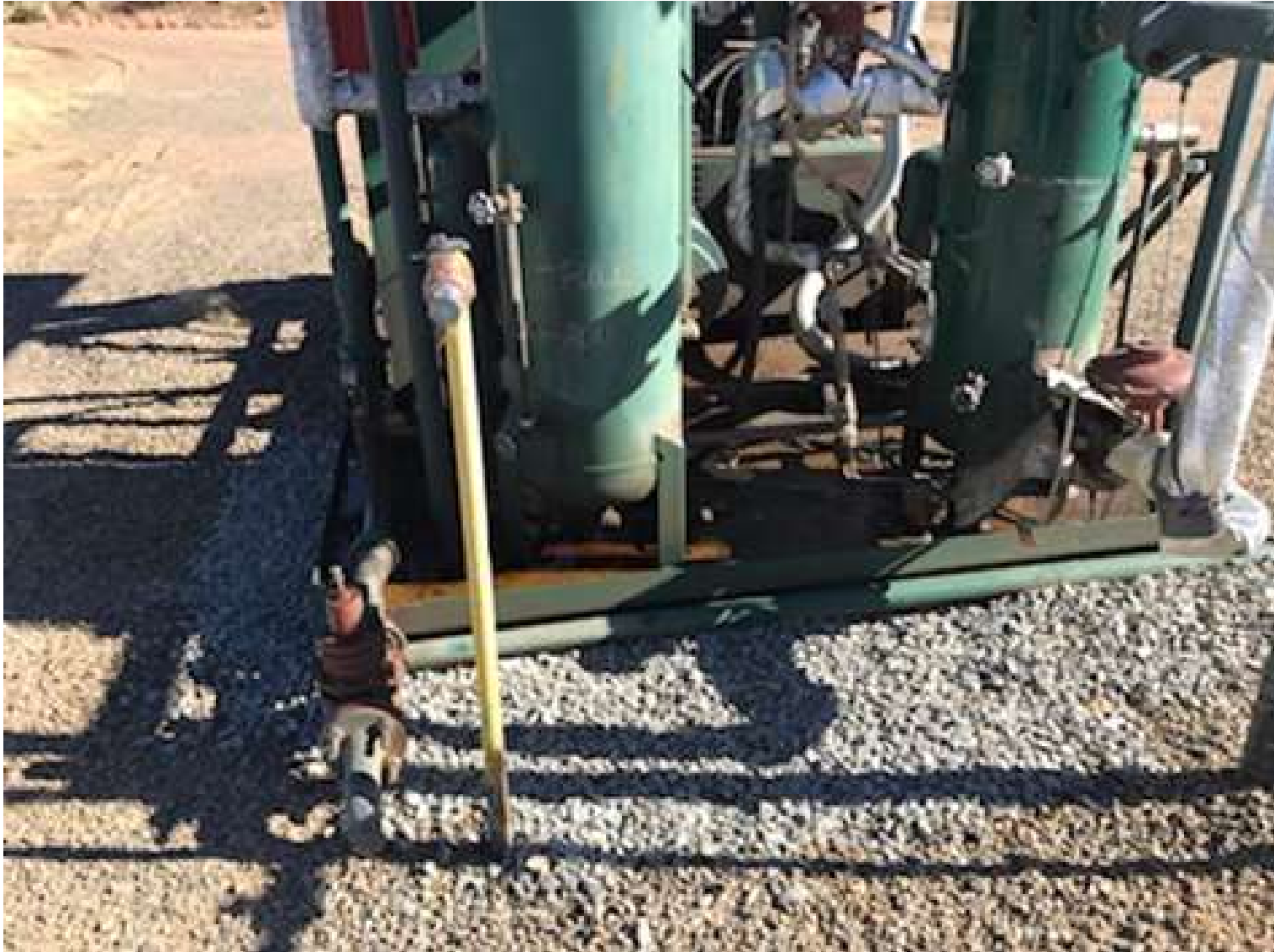
PHOTO 1: THE IMPACTED SOIL NEAR THE LIQUID RING COMPRESSOR WAS REMOVED AND PROPERLY DISPOSED IN ACCORDANCE WITH THE OGRIS OPERATING WASTE MANAGEMENT PLAN.
