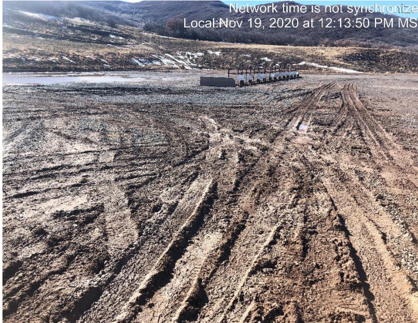
Photo #2283 Sediment is being transported off of location and on to access road.
