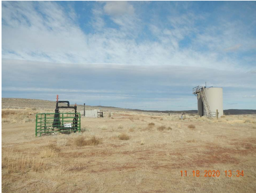
Photo 1. Overview of location taken facing north.
