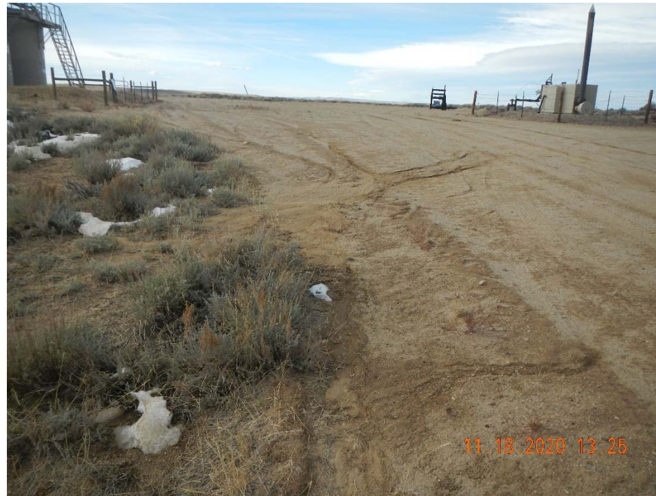
Photo 3. Sediment leaving location at entrance. No stormwater BMPs apparent.
