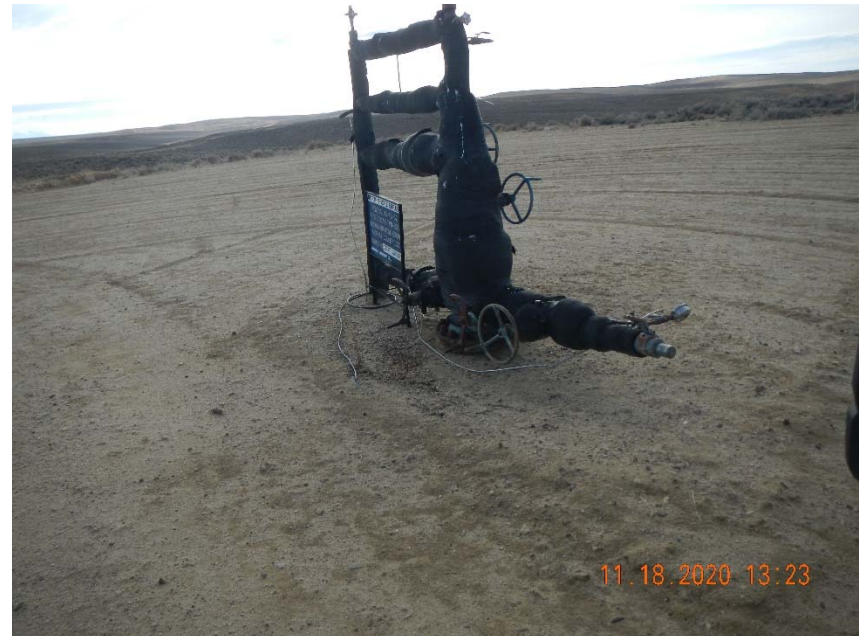
Photo 2. No bradenhead access apparent.
