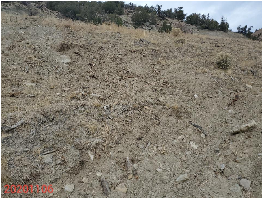
Photo 5: Photo taken from the slopes on the southwest end of the Location. Photo shows erosion observed in inspection #696201578 has been repaired, however no BMPs have been installed to stabilize and protect slopes pursuant to Rule 1002.f.(2)C.
