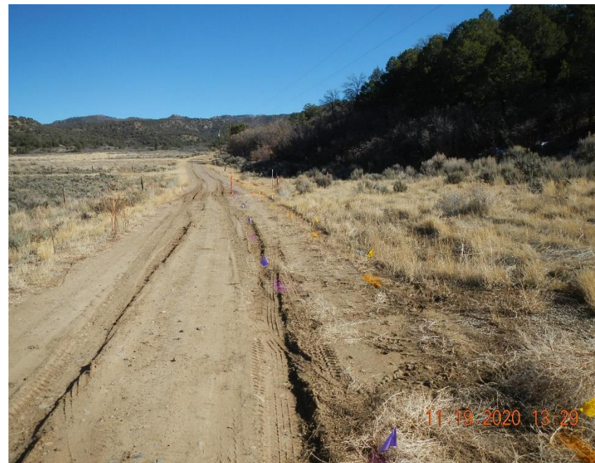
Gas and water flow lines have been marked and release area marked with orange flagging and T posts.
