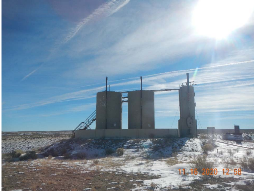
Photo 1. Separator too close to tanks.
