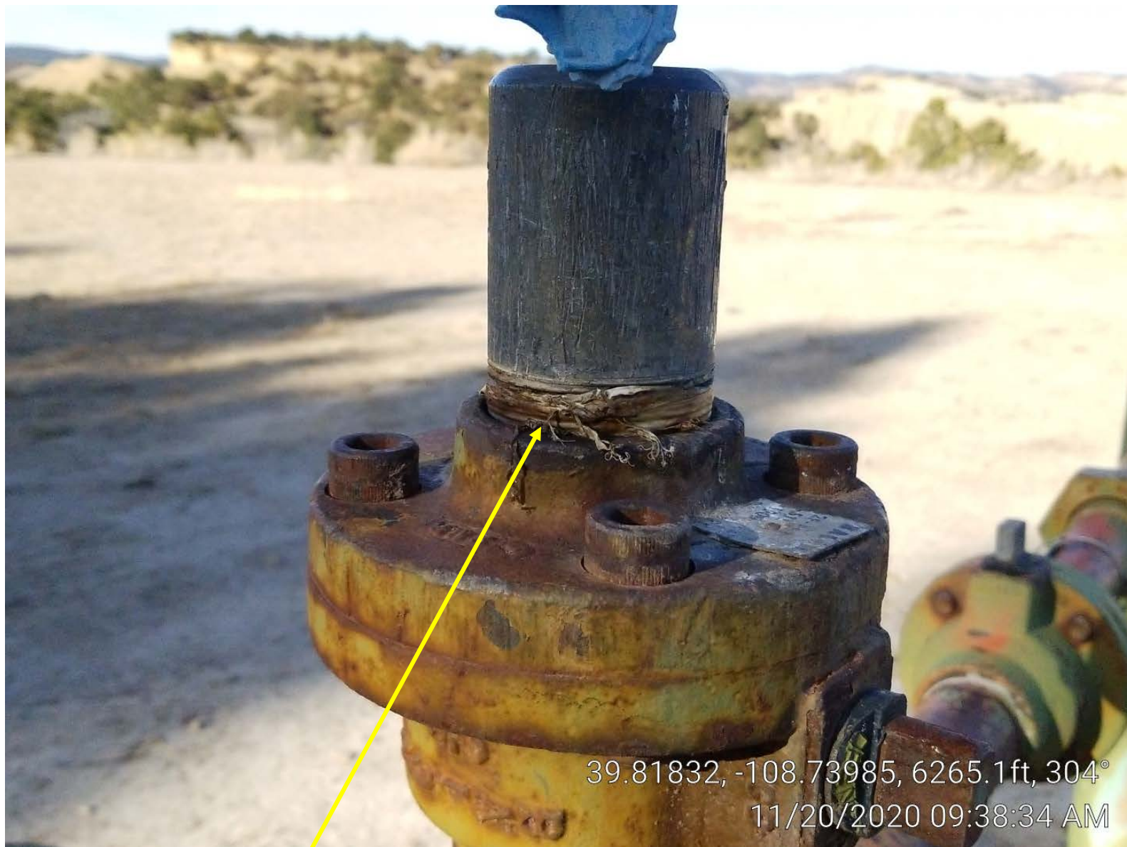
Photo 3. Gas leak.
