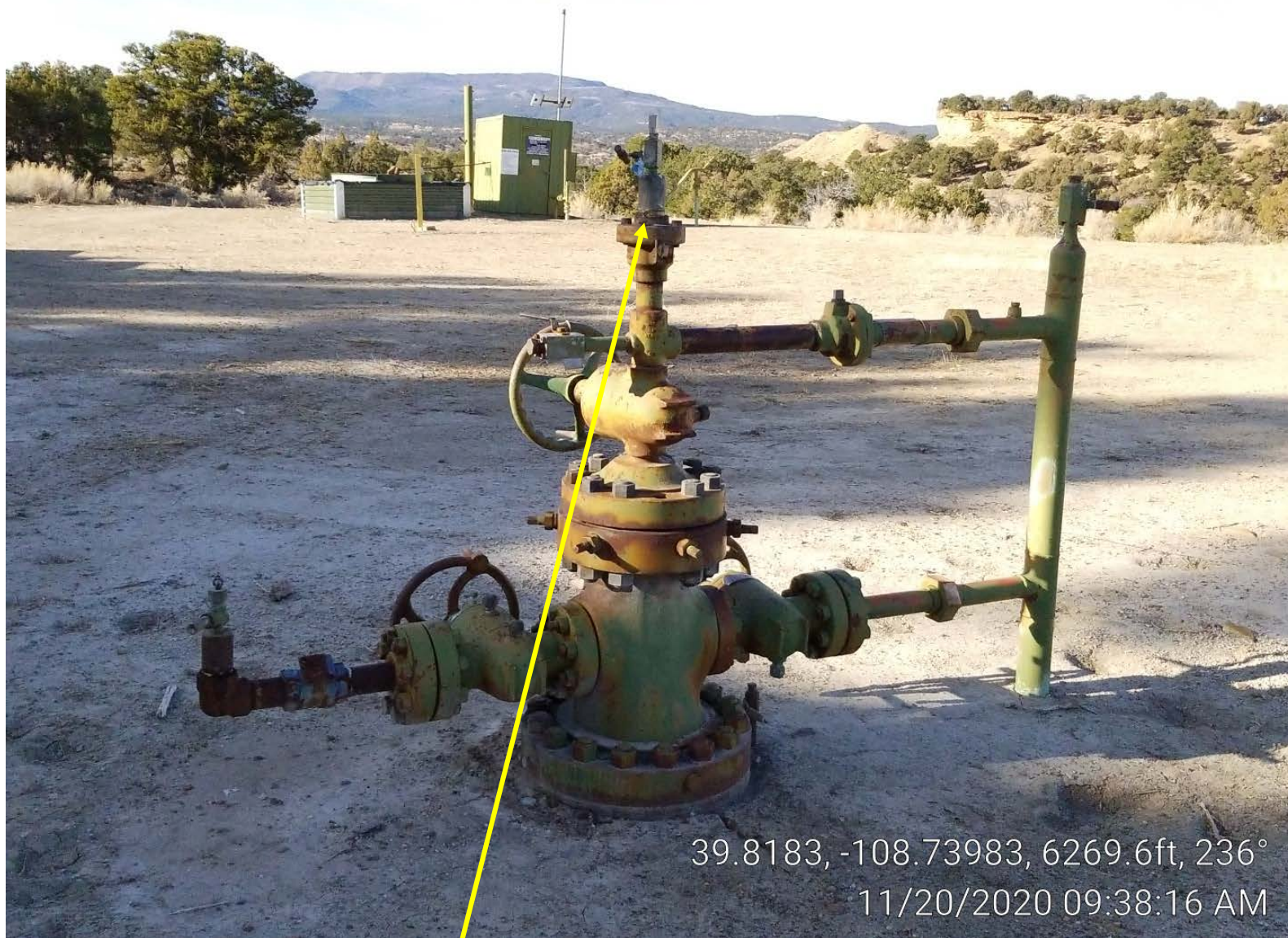
Photo 2. Well with gas leak.
