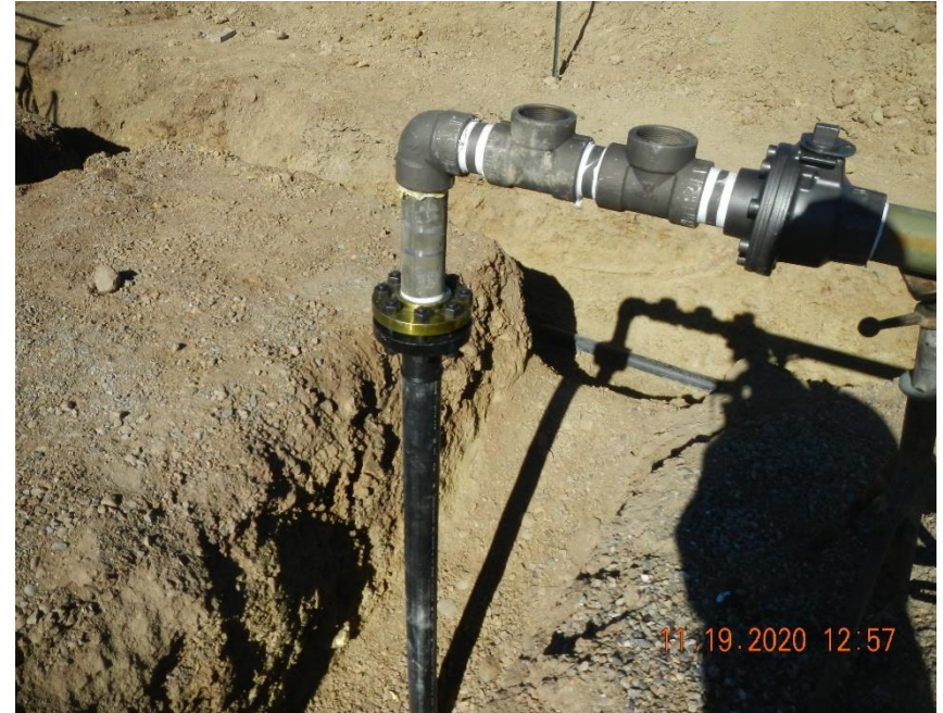
Poly to steel transition upstream of separator.
