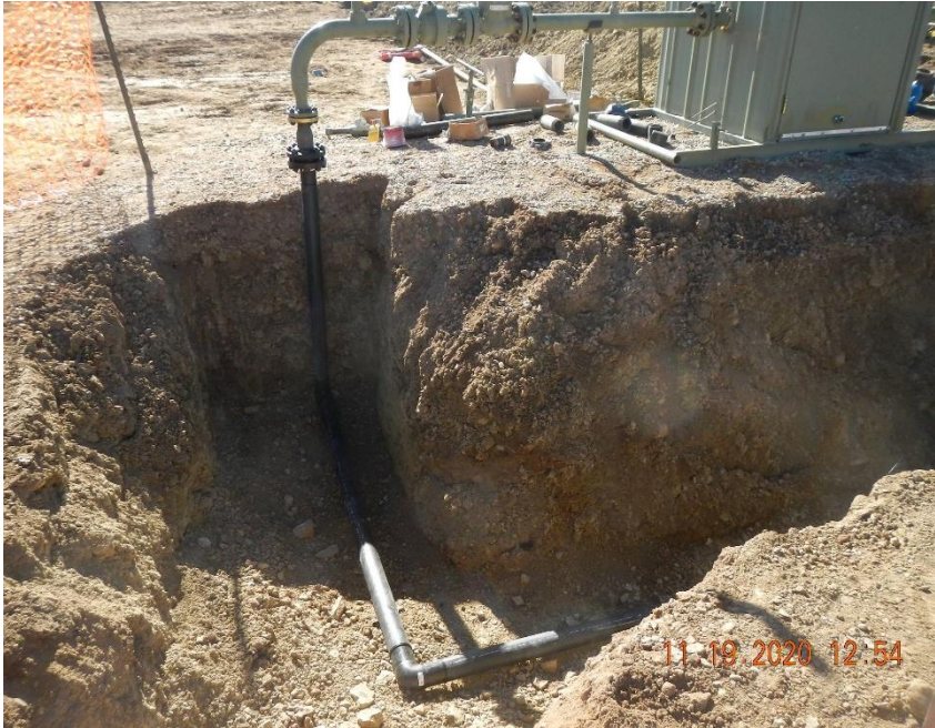
Steel to poly transition at separator.
