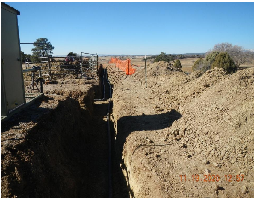
Poly flow lines in open excavation.
