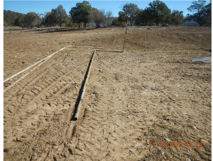
Steel flow lines being replaced with poly pipe.
