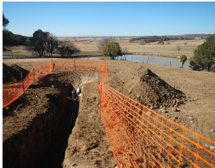
Present termination of newly installed poly flow lines.
