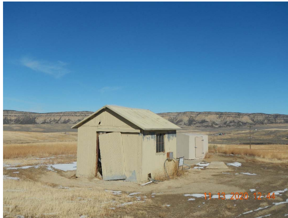
Photo 1. Overview of location taken facing north.
