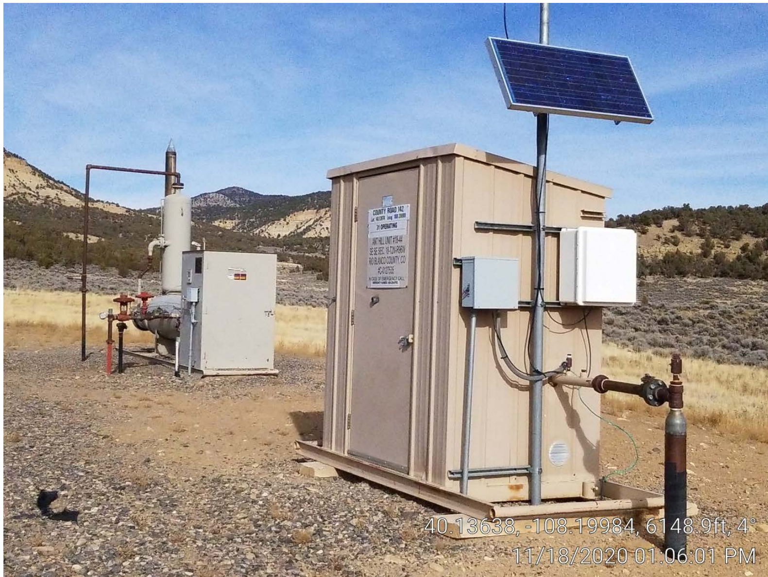
Photo 3. Meter building & separator.
