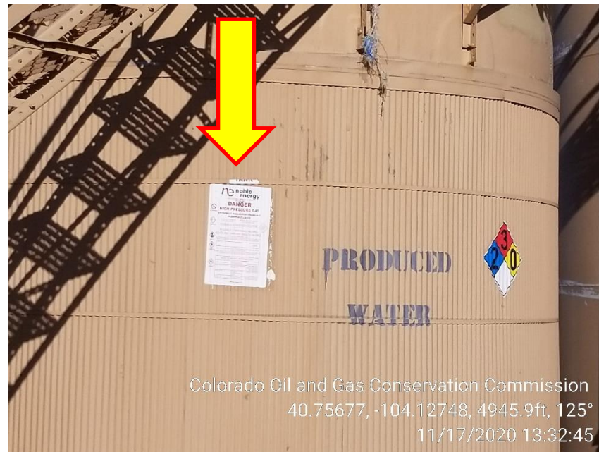
Photo 4 – Produced Water Tank missing Capacity
