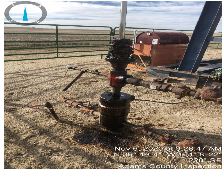
Photo #2 Stained soil around well head
