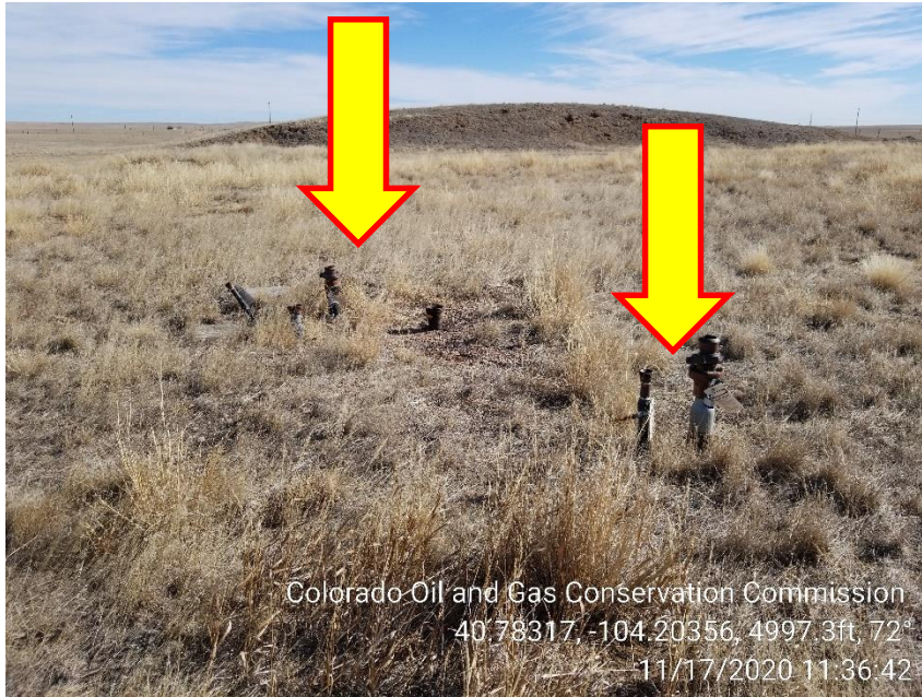
Photo 3 – Unmarked Risers
