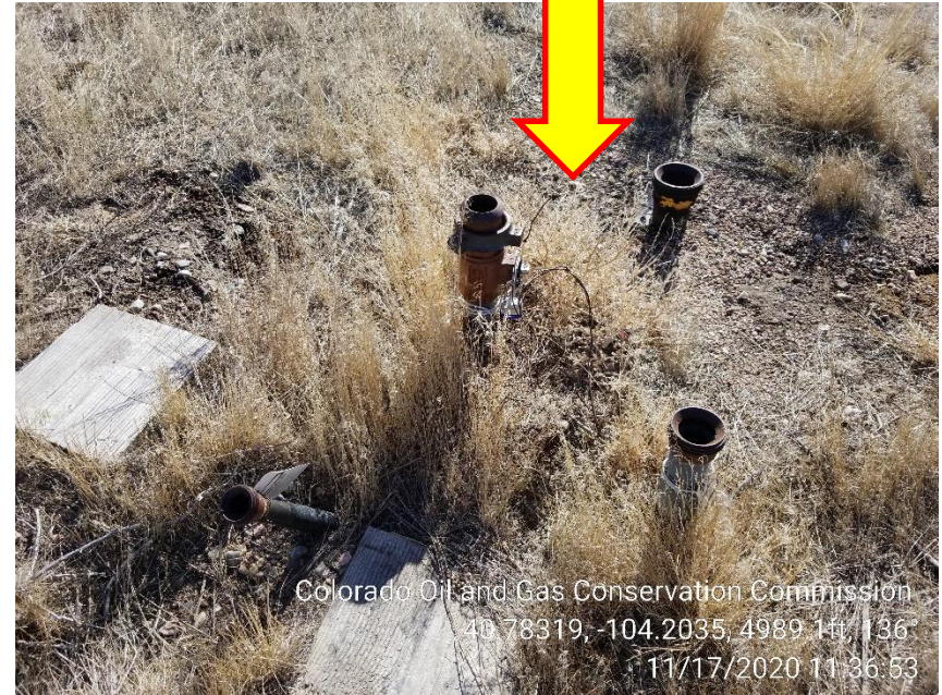
Photo 4 – Unmarked Risers
