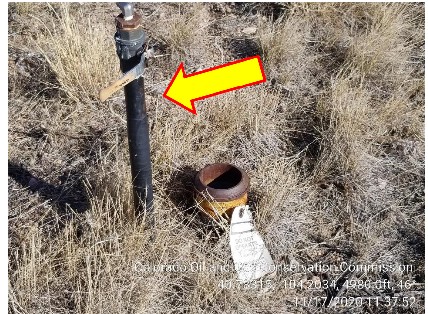
Photo 6 – Unmarked Risers
