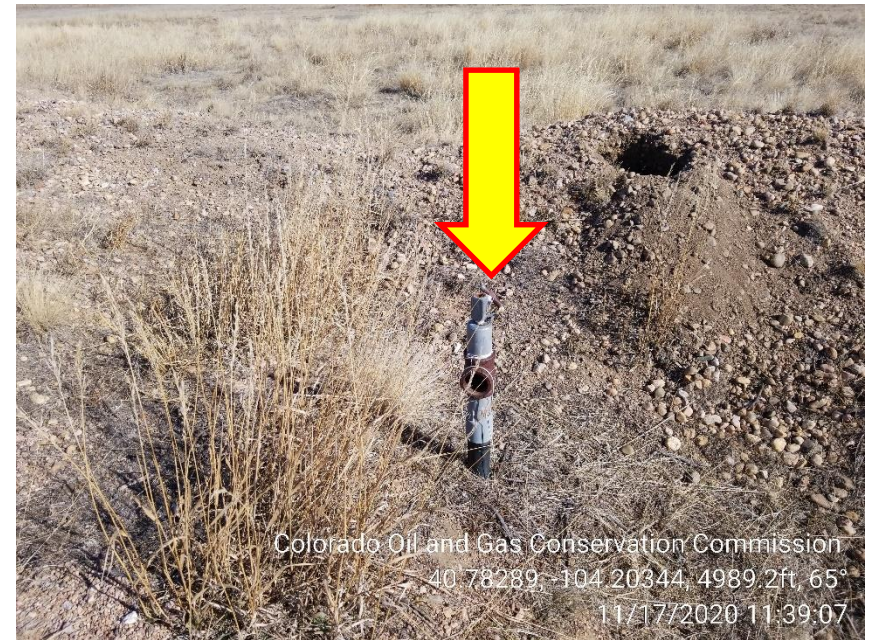
Photo 10 – Unmarked Riser
