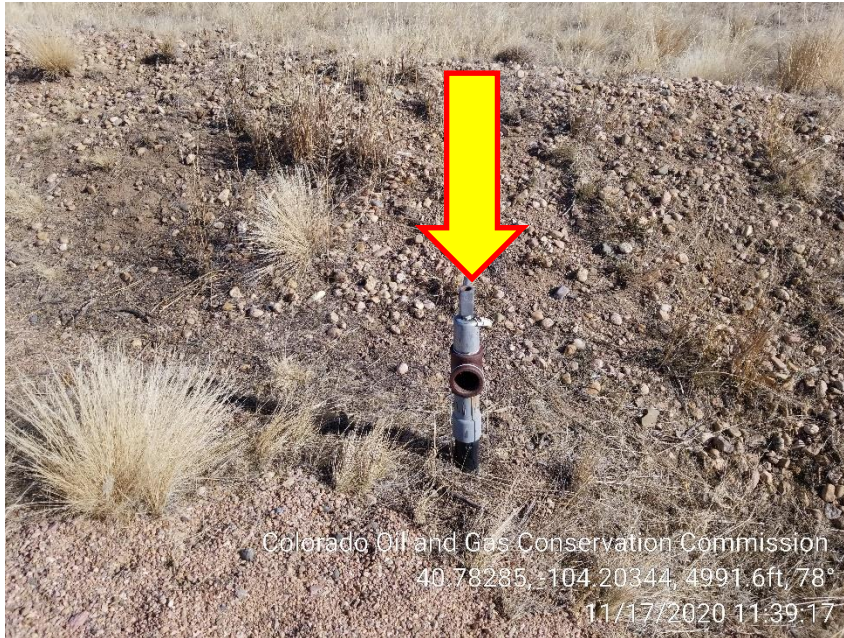
Photo 11 – Unmarked Riser
